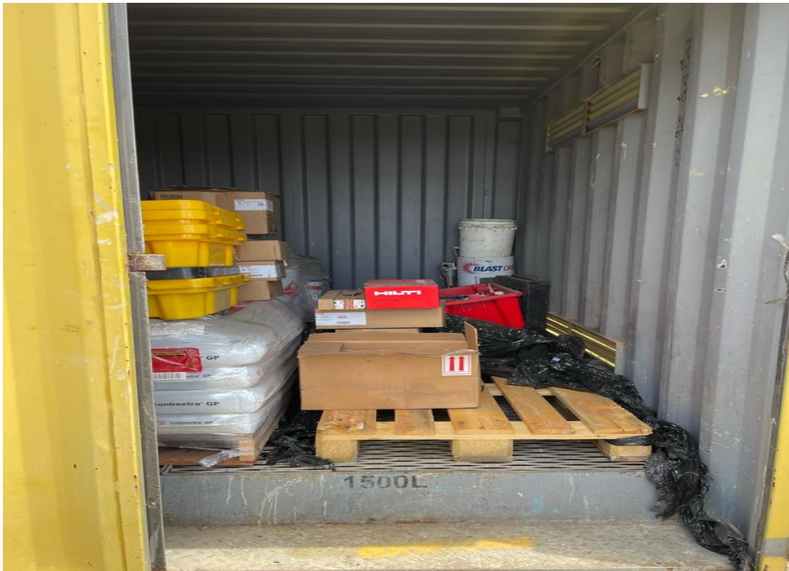
Plate 1 Bunded chemical storage area
