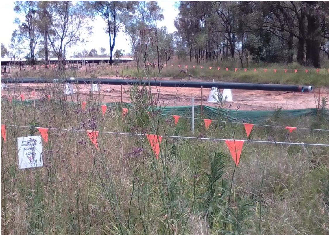
Plate 11 Above ground pipeline section
