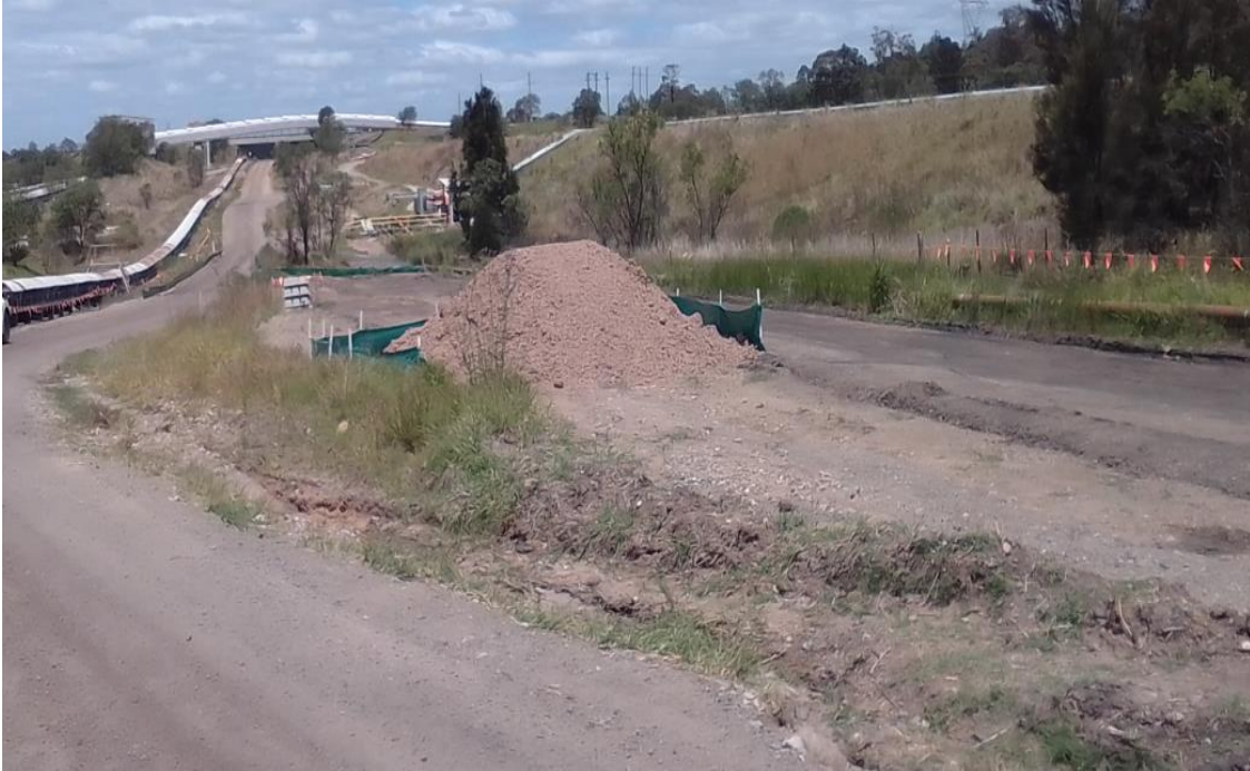
Plate 9 Sediment fences used around stockpiles
