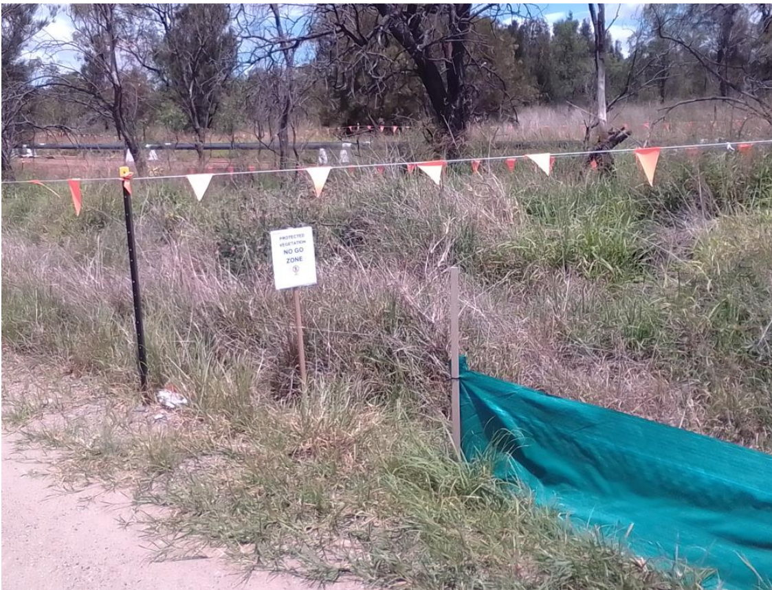
Plate 10 'No-go' signage for protected vegetation
