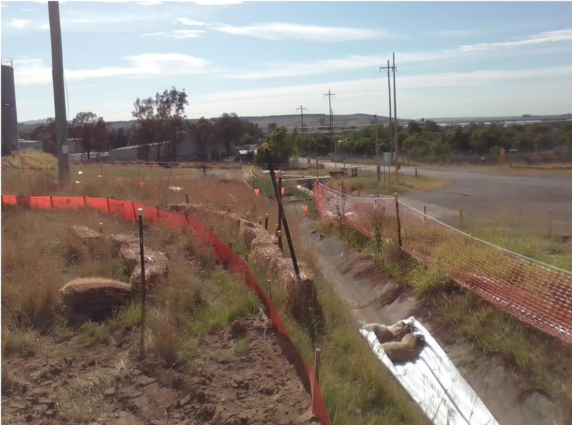
Plate 5 Sediment mitigation measures in place for the project construction area
