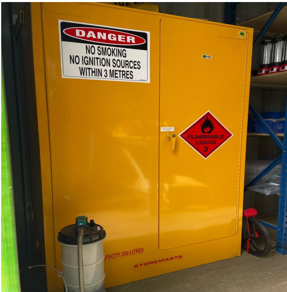
Plate 2 Chemical Storage Cabinet available at project laydown area
