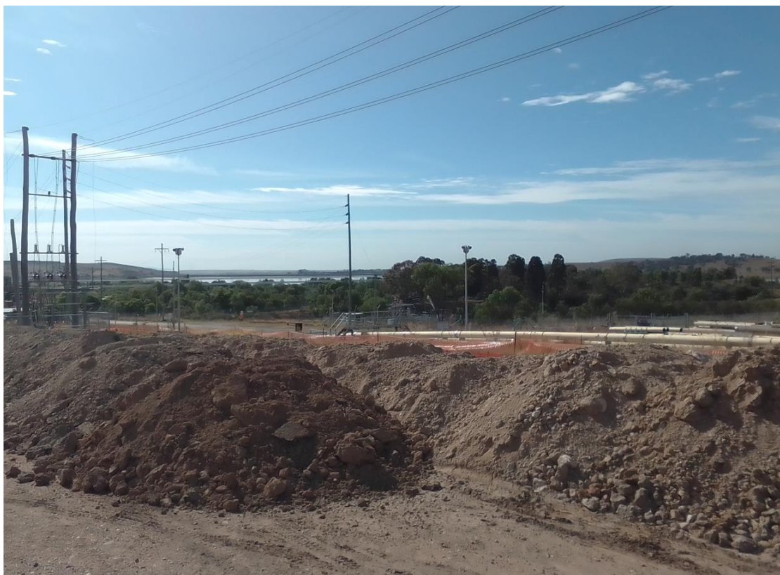
Plate 10 Stockpiles at project construction area with sediment fencing in place
