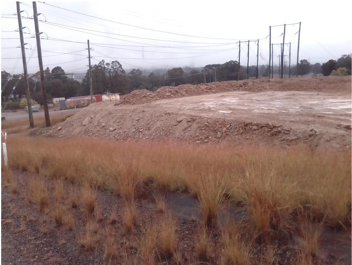
Plate 13 Excavated materials stockpile adjacent project construction area
