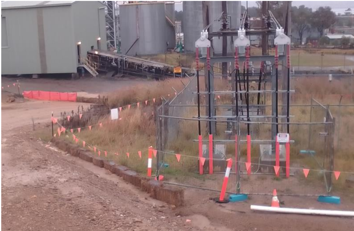
Plate 5 Sediment mitigation measures in place for the project construction area
