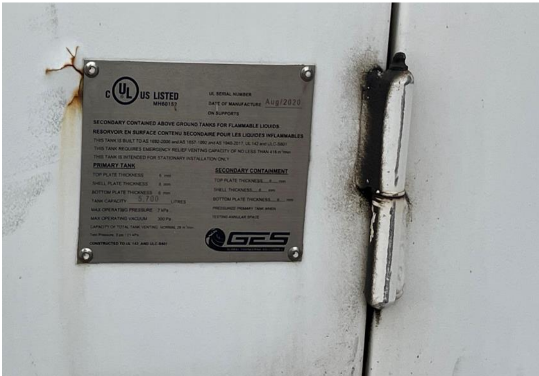
Plate 5 5,700 L Diesel secondary containment tank available on site
