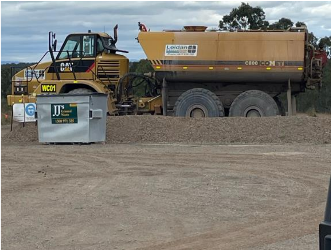
Plate 12 General waste skip bin available on site
