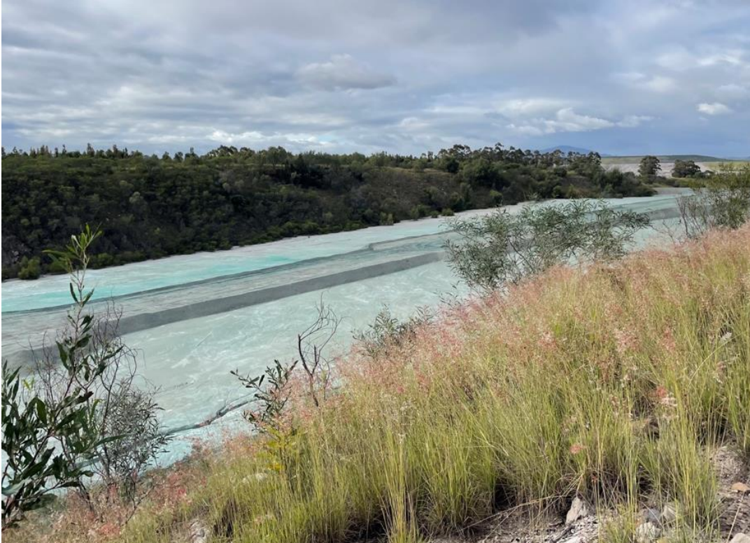
Plate 3 Polymer dust suppression used on Void 5
