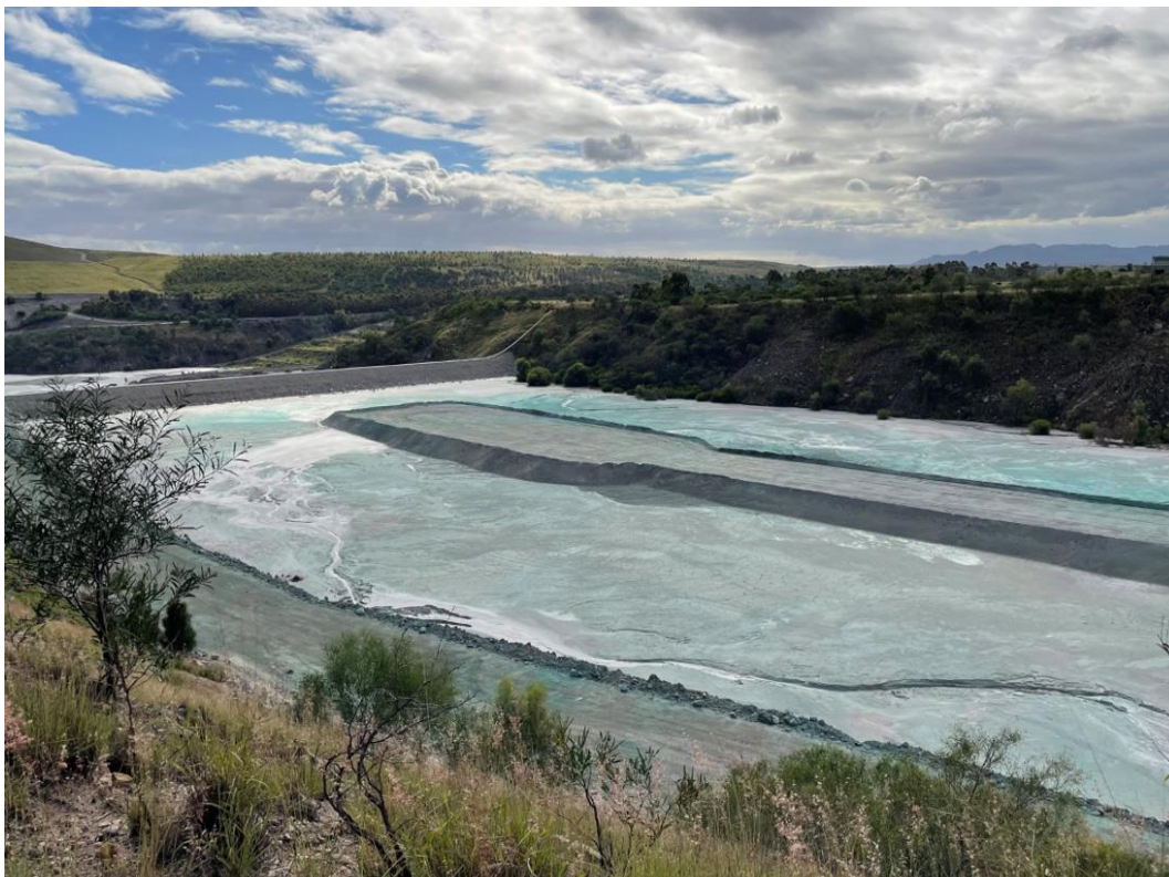
Plate 2 Polymer Dust Suppression used on Void 5
