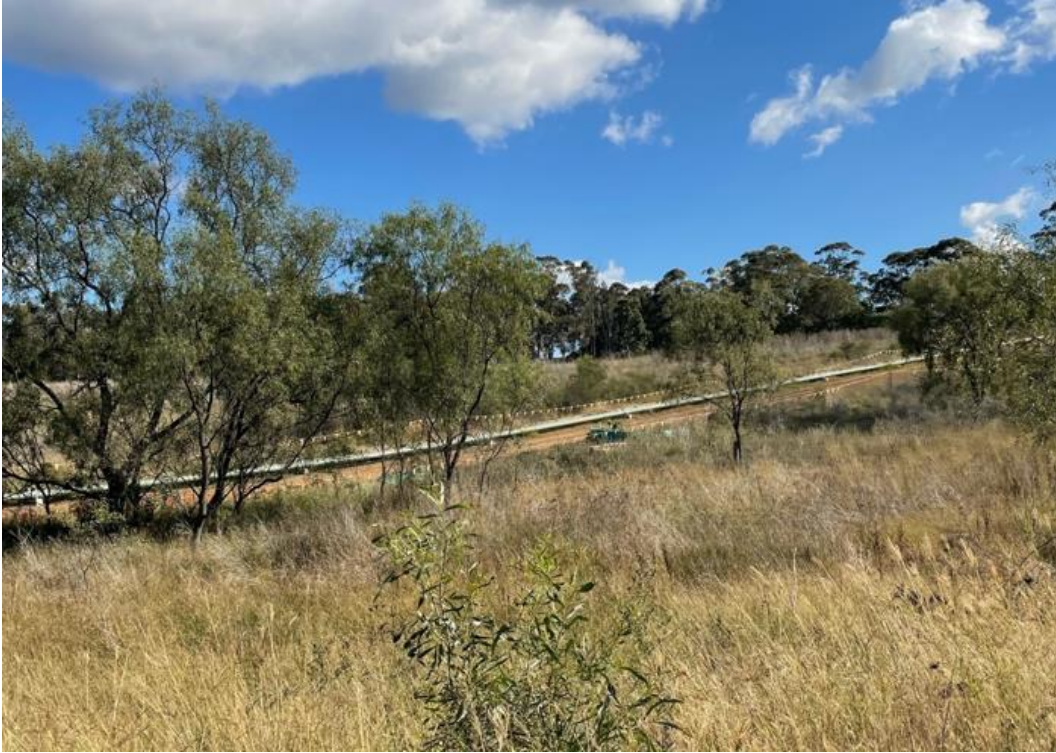
Plate 11 Above ground pipeline section
