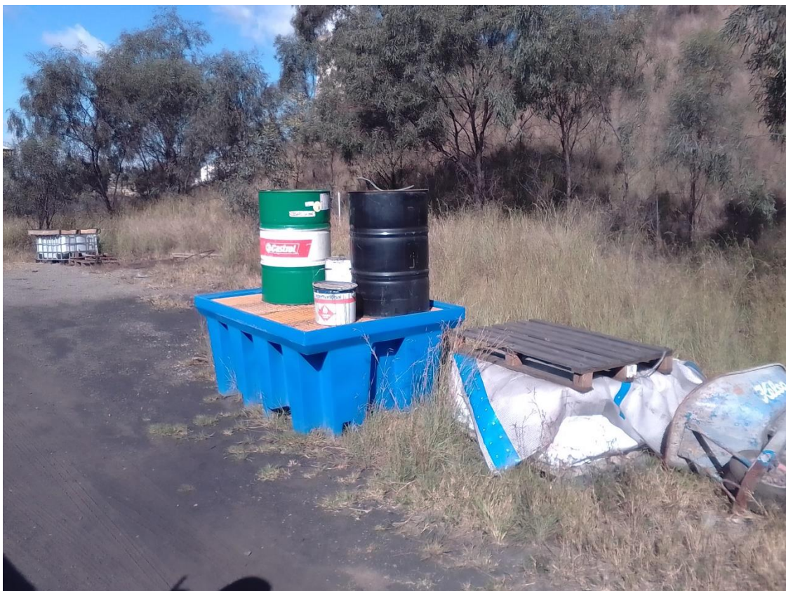
Plate 2 Waste chemicals / oils stored on bunded pallet at project laydown area
