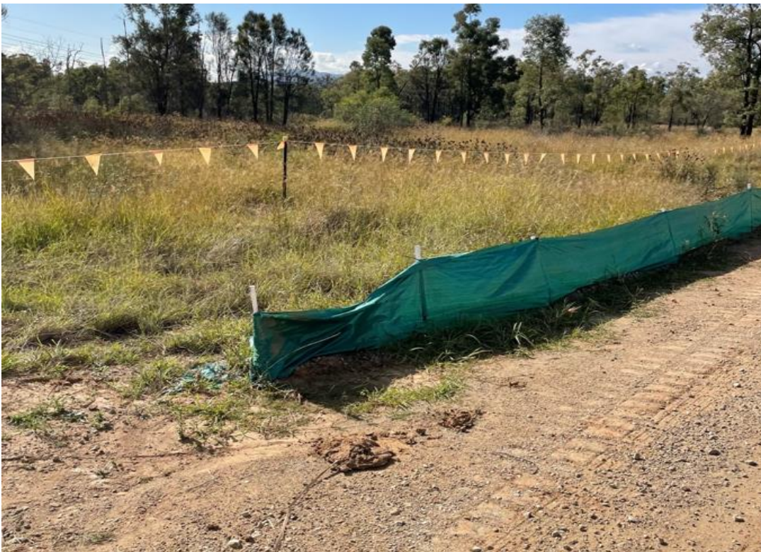
Plate 12 Sediment control and flagged project disturbance boundary
