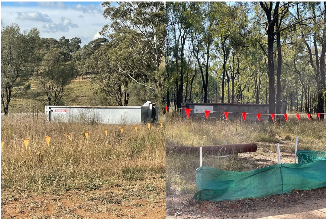
Plate 14 Waste skip bins located outside of flagged project area
