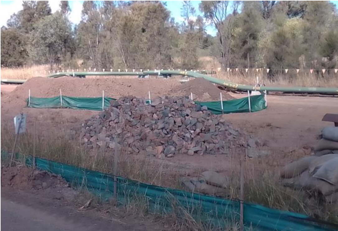
Plate 9 Sediment fences used around stockpiles
