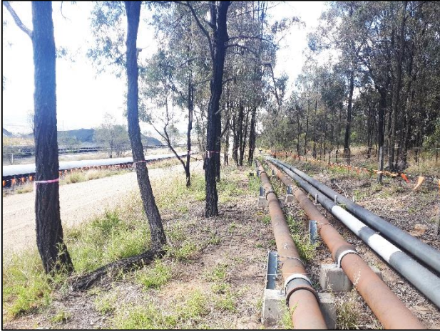
Plate 1: Demarcated trees to be removed next to the existing ash line
