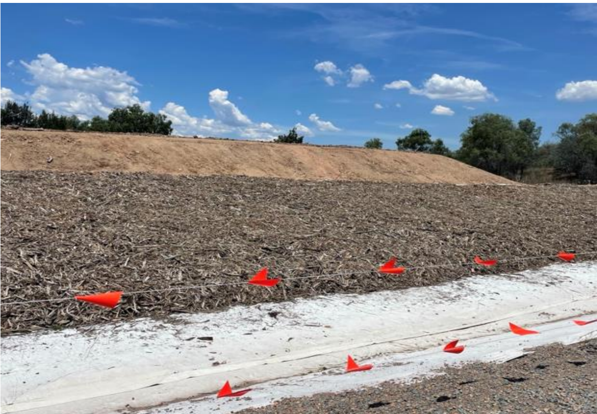
Plate 12 – Flagging and sediment control for Stage 2 of the Project
