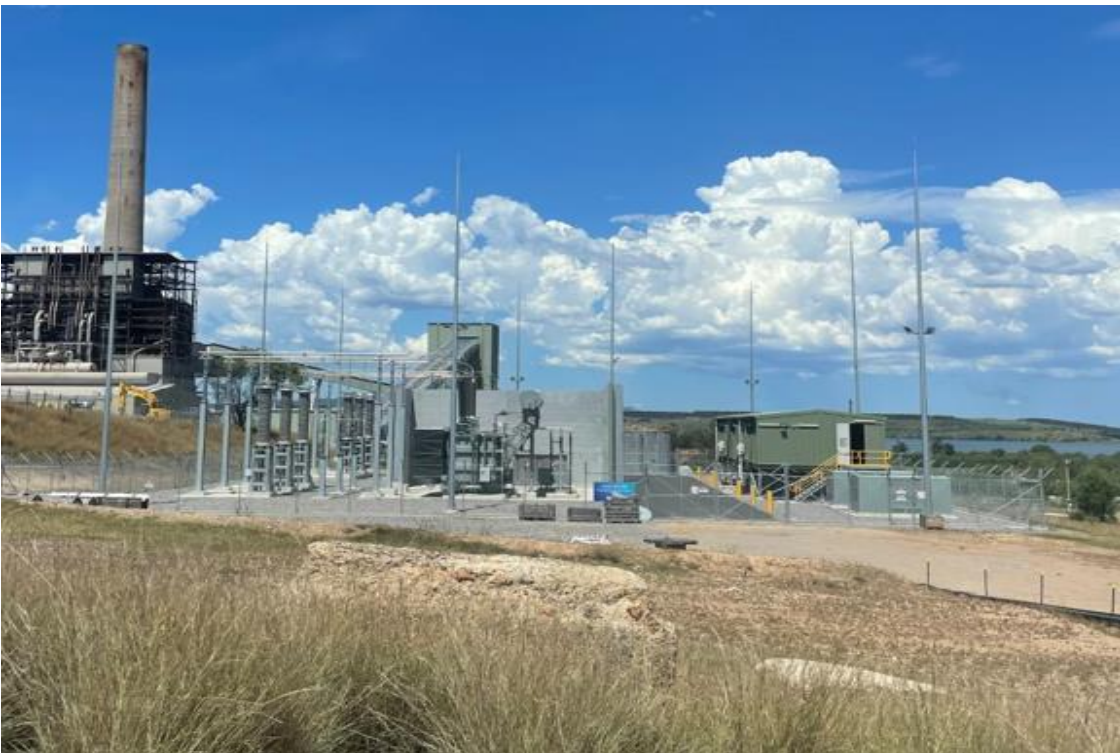
Plate 18 – Completed Stage 1 Project area
