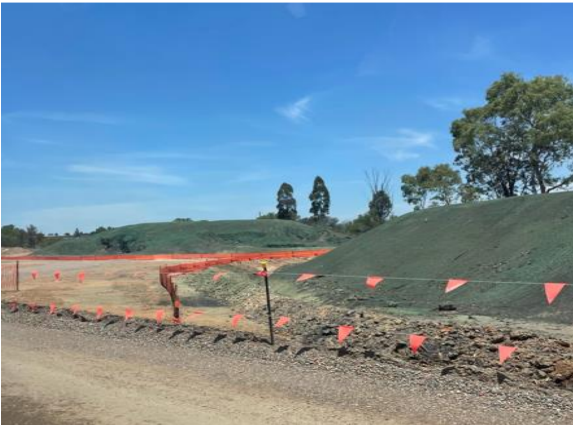
Plate 4 – Hydromulch used on Stage 2 stockpiles for dust suppression
