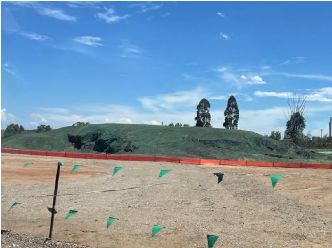
Plate 5 – Hydromulch and sediment fencing being used around Stage 2 stockpiles
