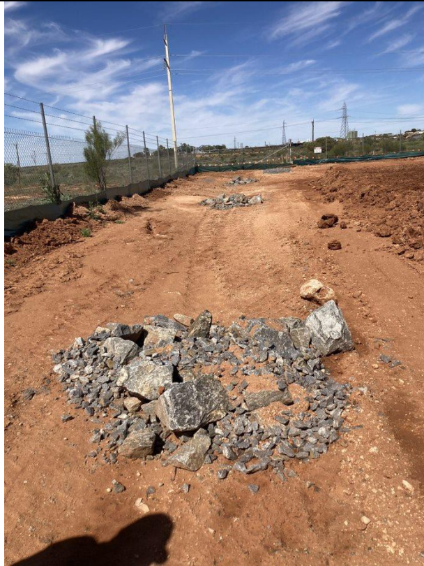
Water drainage controls on construction pad.
