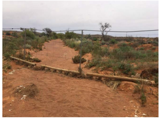
Plate 22. Fence repairs made in May 2021
