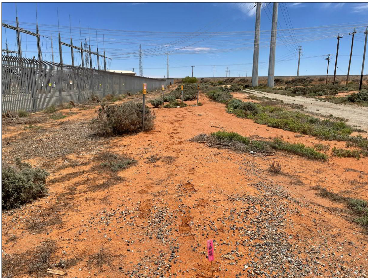
Plate 3 View northwest showing disturbance adjacent to the Transgrid substation (source: AECOM 2021)
