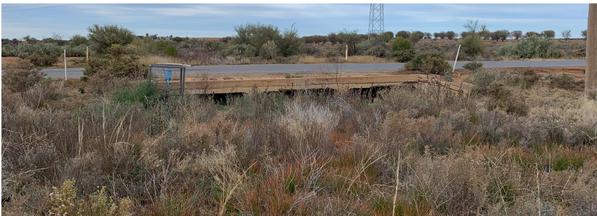
Figure 3 Culverts passing under Pinnacles Road
