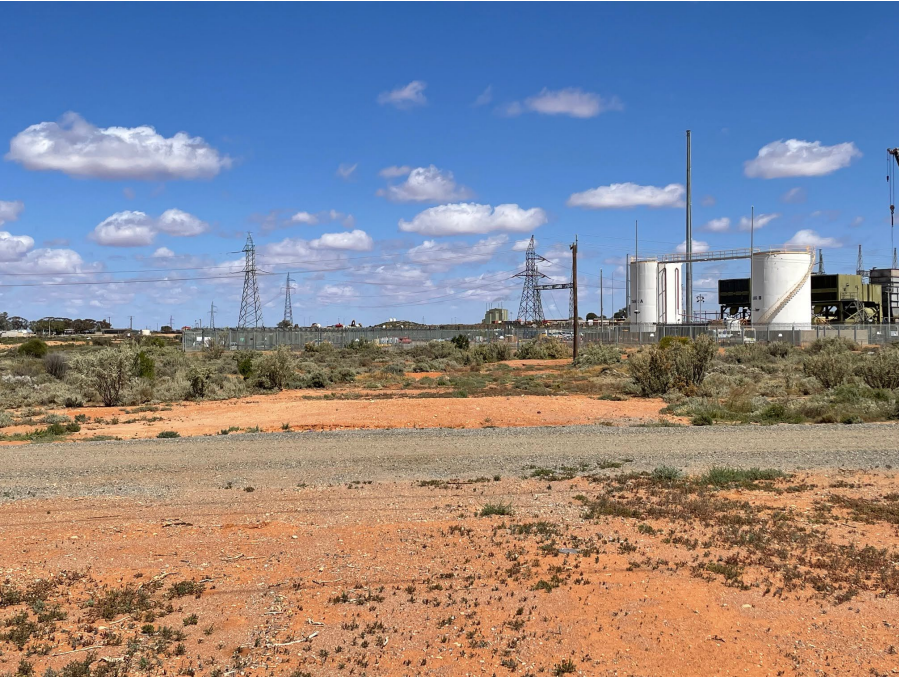
Photo C10: High voltage transmission connection (underground)
