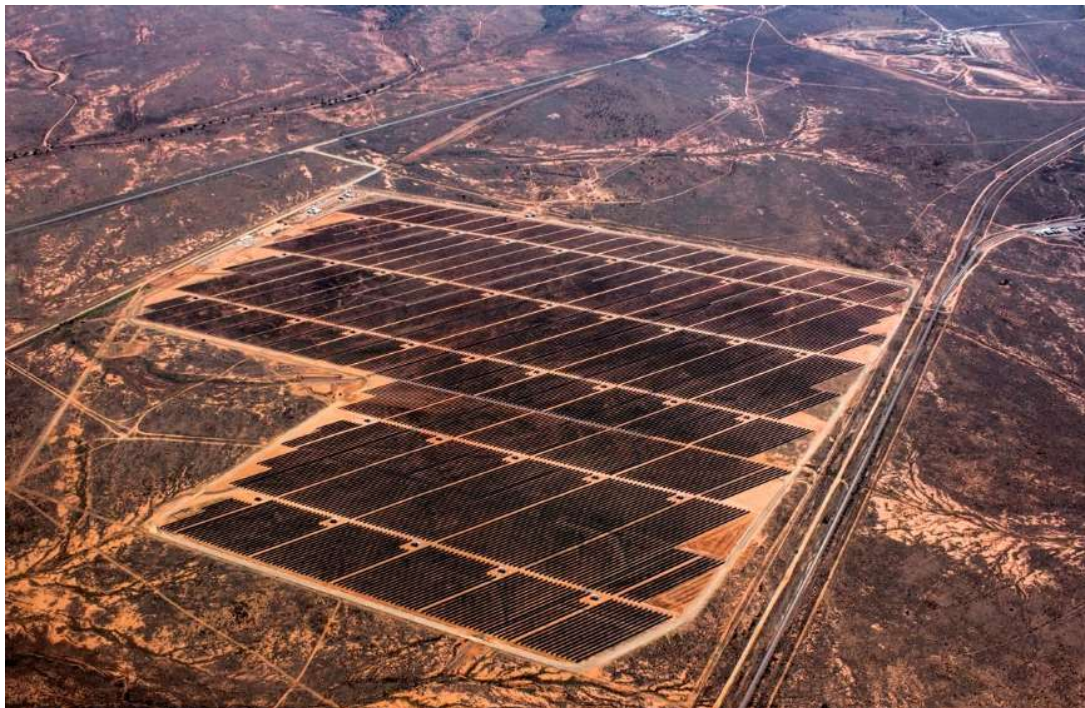
Figure 2. Aerial Image of BHSP (Nov 2015) Aerial image shows the BHSP with site access from the Barrier Highway, and the overhead line across Willyama Common to the East.
