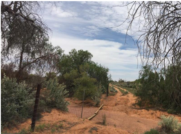
Plate 21: Fence repairs made in May 2021
