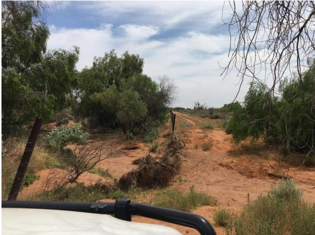
Plate 19: Damaged fence observed in 2020
