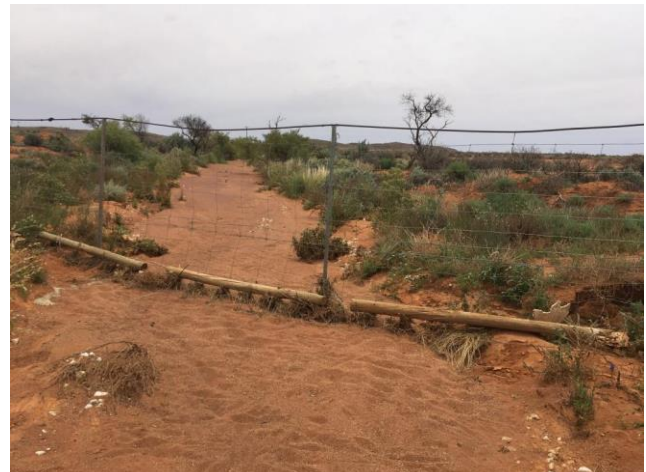
Plate 22: Fence repairs made in May 2021
