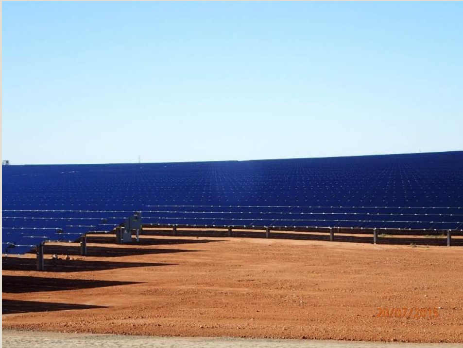
Module installation complete
