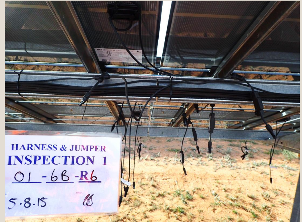
Quality inspection - above ground cable installation
