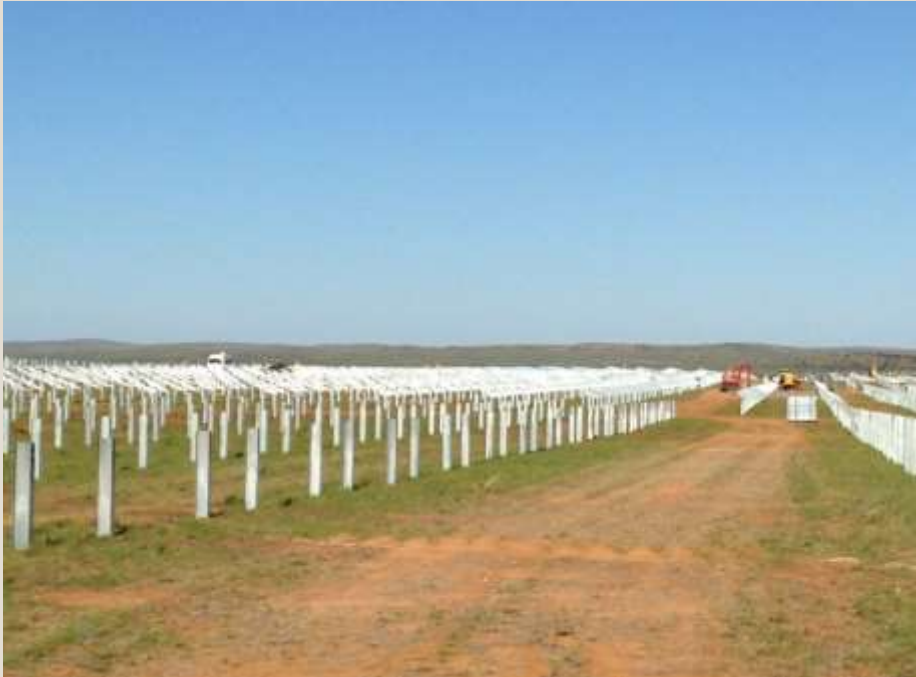
Post and tilt installation
