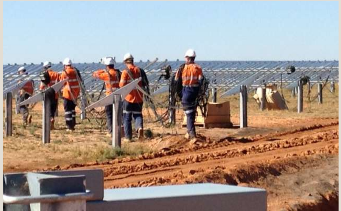
Above ground cable installation
