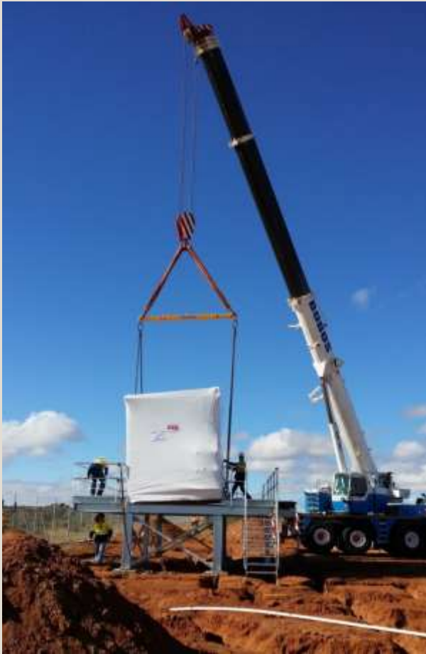
Lifting switchgear into position
