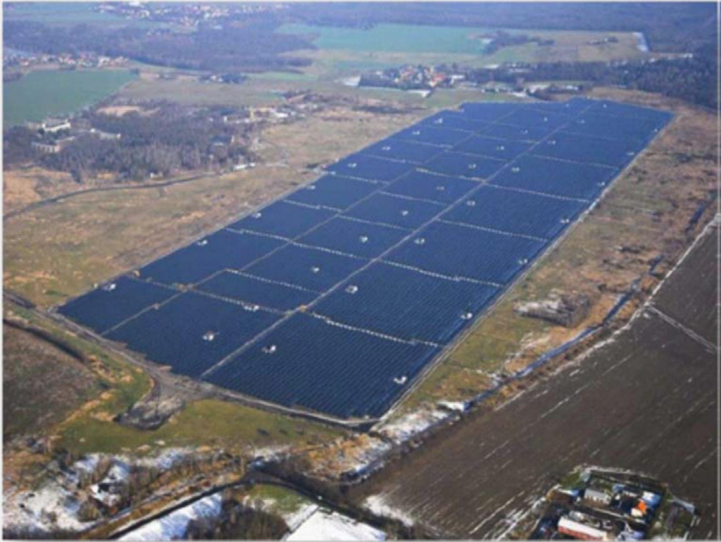
Figure 5-3 An example of a 40 MW plant in Germany
