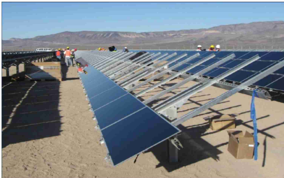
Figure 4 Photovoltaic modules and brackets under construction
