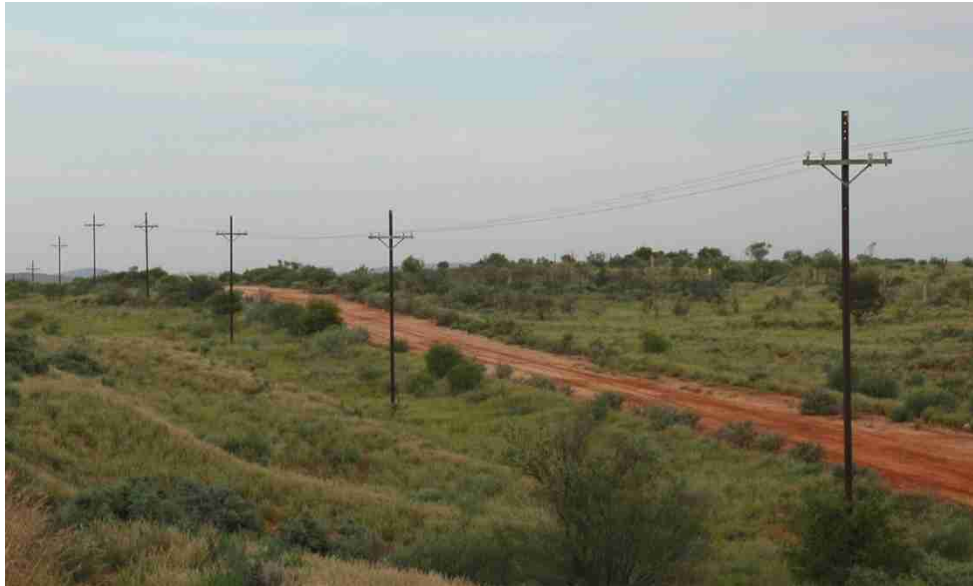
Figure 9 Existing transmission line adjacent to the solar project site.
