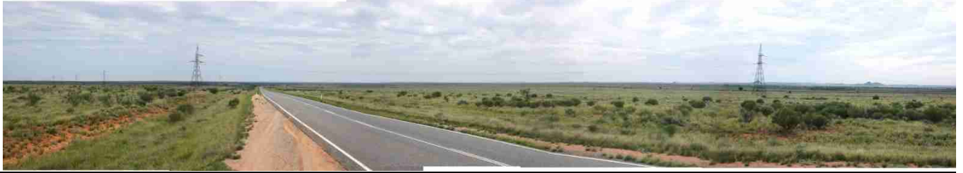
View southeast toward crossing point of existing 220kV transmission line
