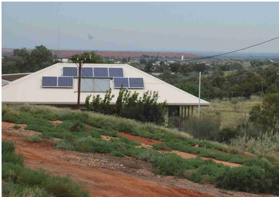
Figure 11 Residence adjacent to Lunam Street with roof mounted solar panels.
