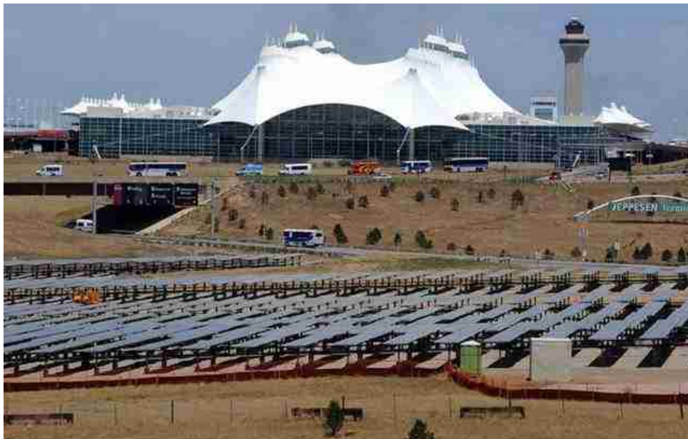
Figure 55 Denver International Airport Solar Project.
