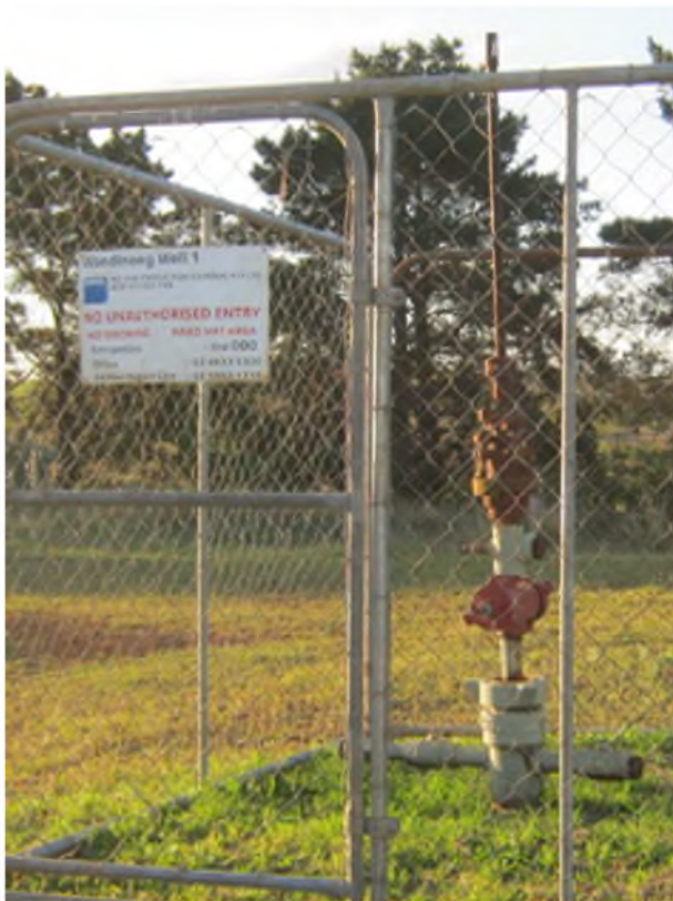
WG01 Prior to Cut and Cap
