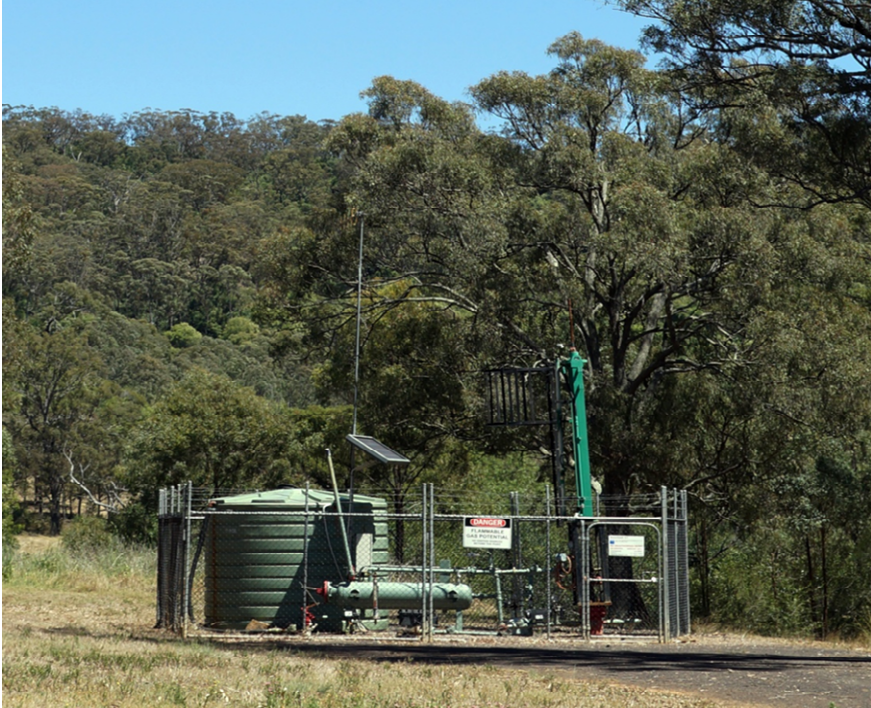
Gas well with Pump and Water Tank
