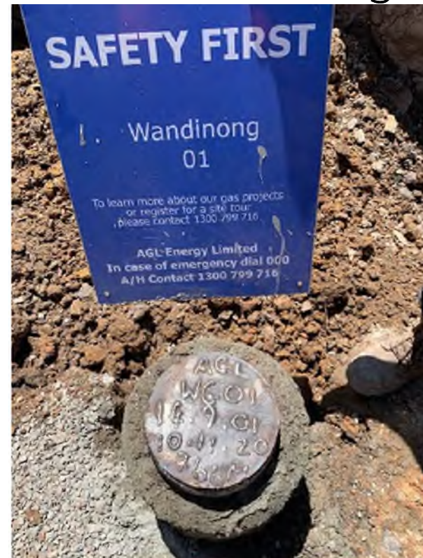
WG01 Well Head P&A Plate installed
