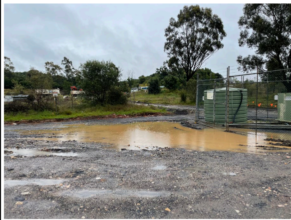
Photo 9: Well site GL02 (rehabilitation in progress). Well site GL02 is co-located with well site GL12 which is operational
