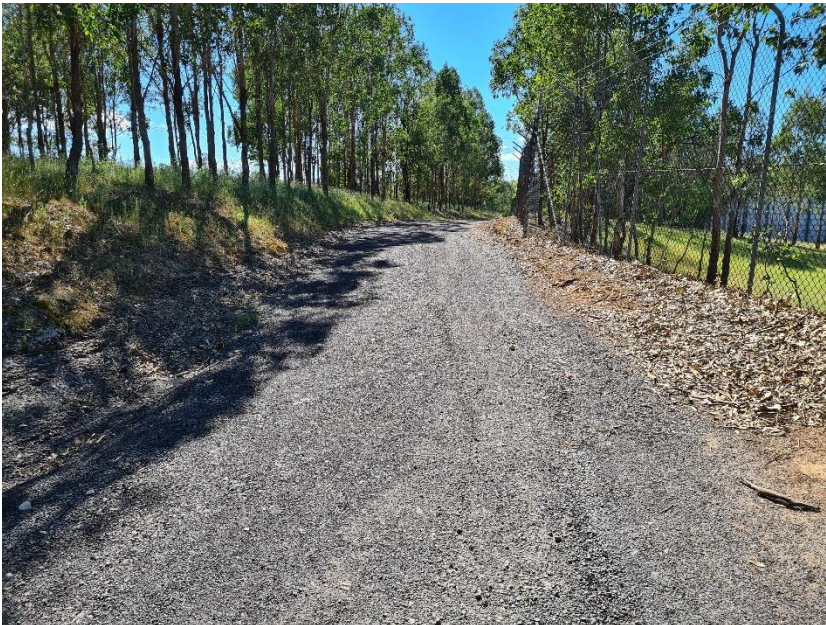
Photograph 3.4 Native trees on internal access road cut batter
