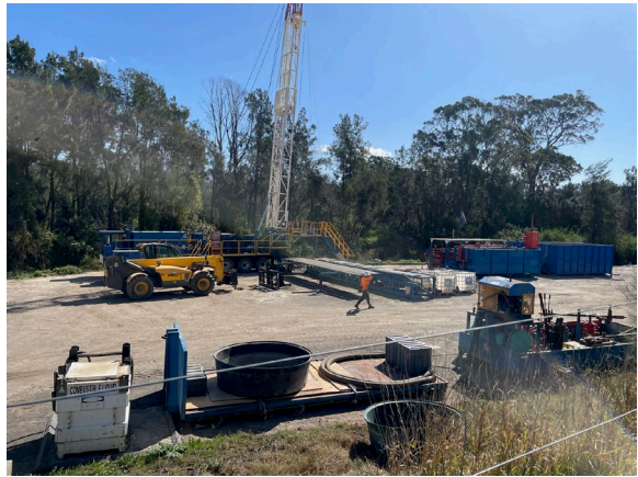
Photo 12: Well site MP16/MP25 (decommissioning in progress)
