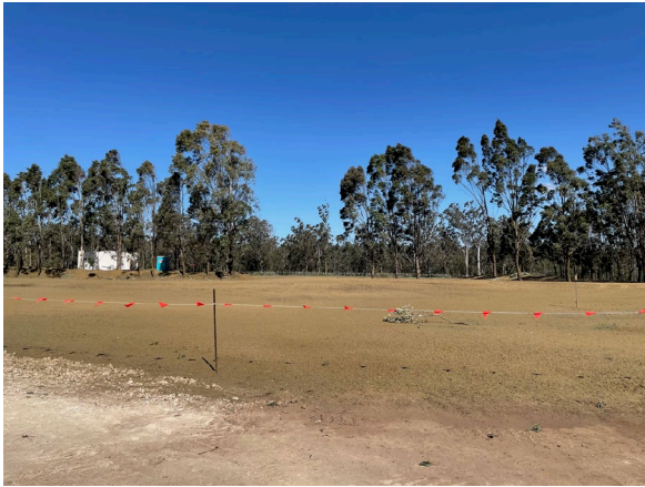
Photo 9: Rosalind Park Gas Plant (rehabilitation in progress)
