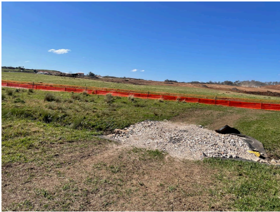
Photo 11: Piped creek crossing
