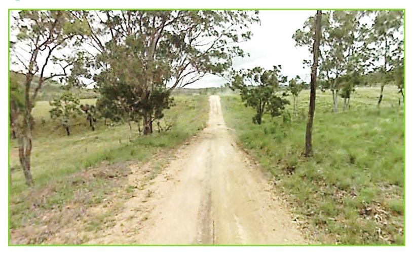
Sections of Niagara Road have steep, undulating gradients which make heavy vehicle passage difficult.
