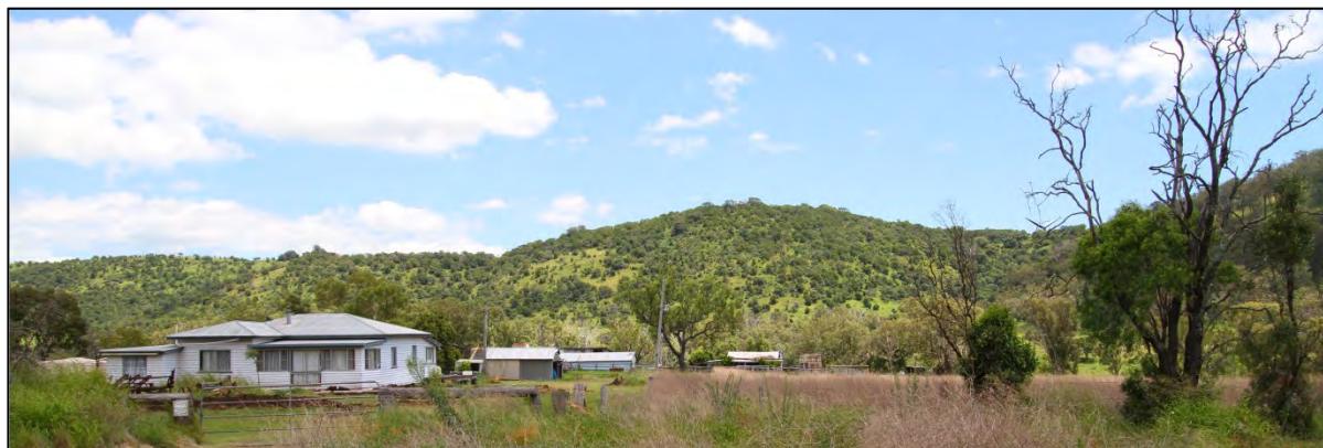
Photomontage view from Viewpoint 8: Northerly view from the Bunya Highway (75° field of view)
