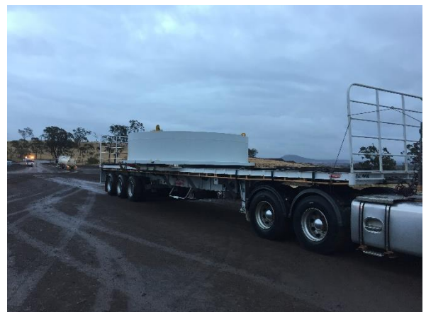
Wind turbine base ring delivery to site
