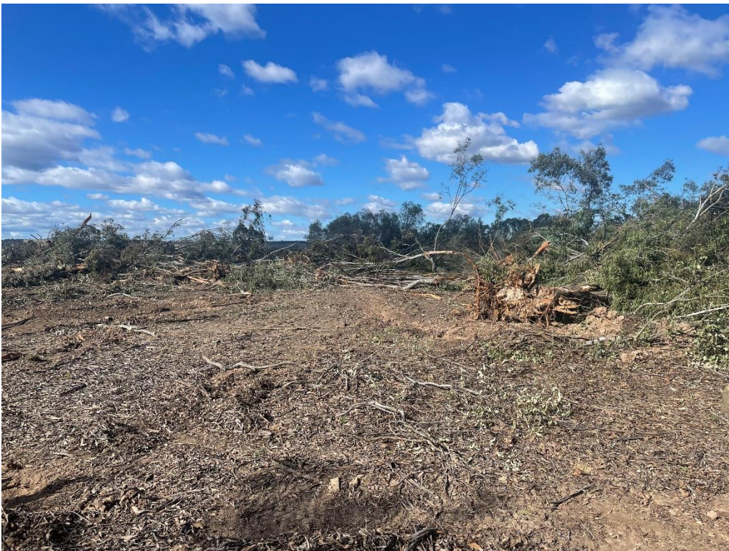
Plate 14 Cleared vegetation stockpiles within Stage 2 disturbance boundary
