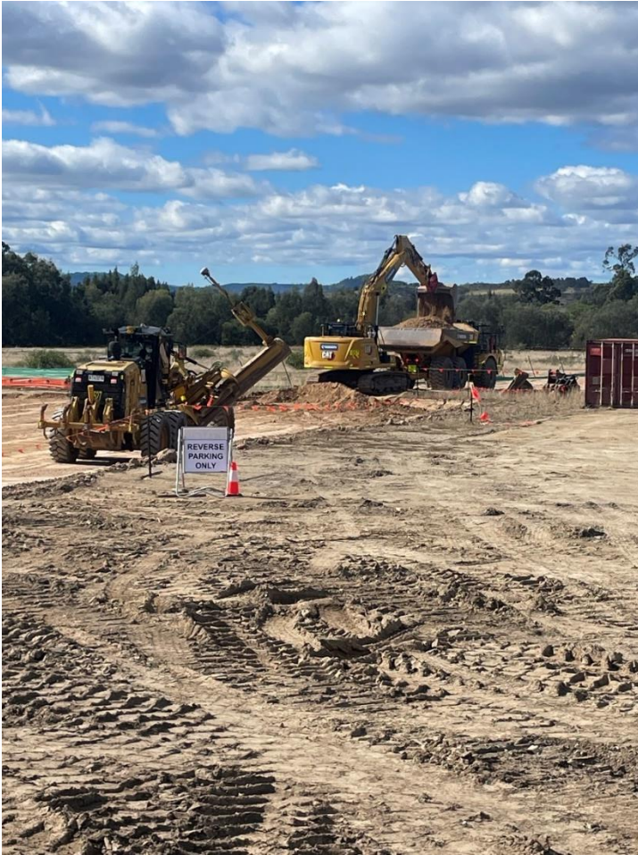
Plate 9 Truck loading with controlled drop heights. Minimal dust generated by vehicle movements
