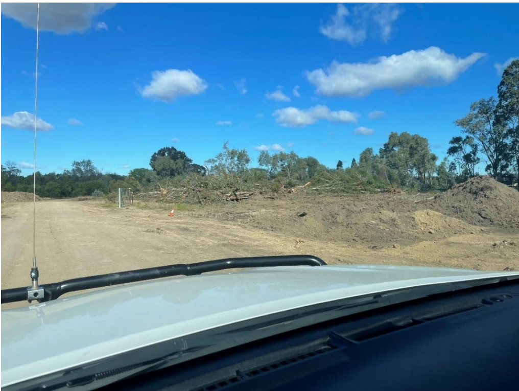
Plate 10 Cleared vegetation stockpiled within Area 2, Stage 2
