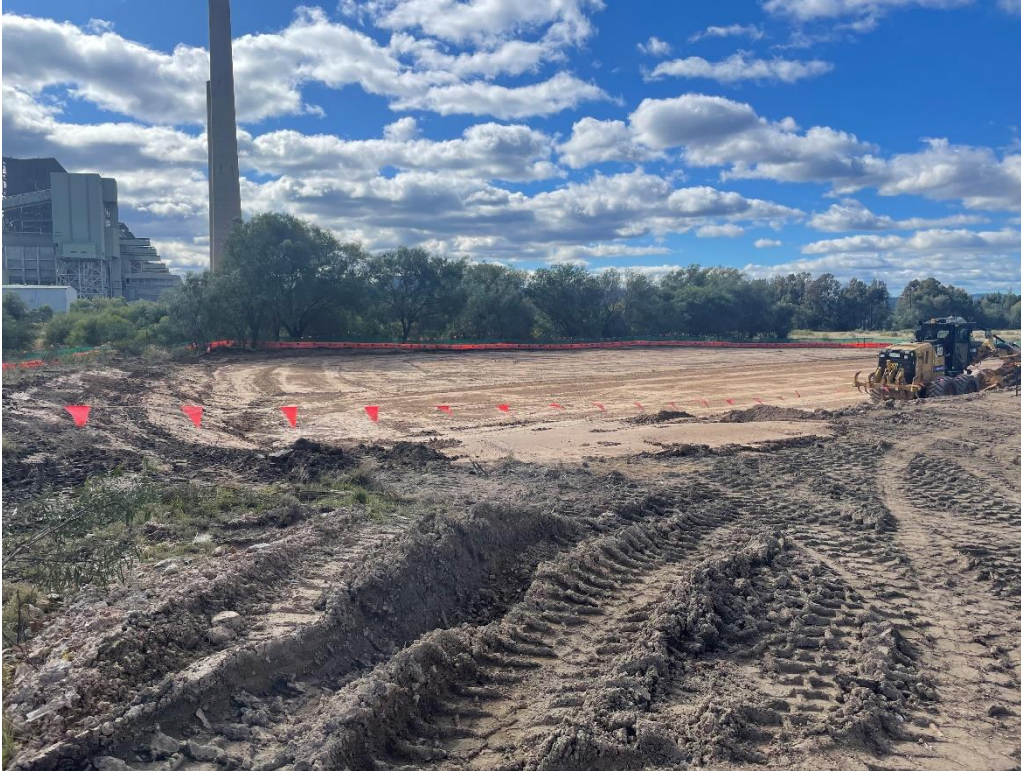
Plate 13 Stage 2 construction area, showing no signs of elevated dust
