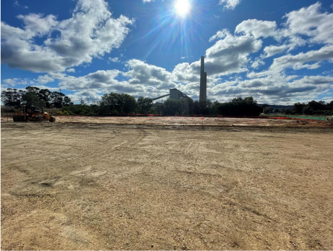
Plate 3 Area 2, Stage 2 disturbance preparing area for BESS installation
