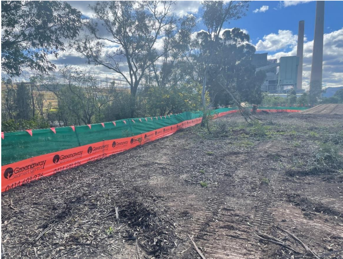
Plate 5 Area 2, Stage 2 sediment fencing and disturbance boundary delineation
