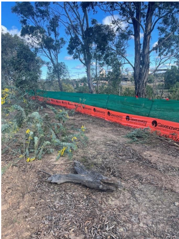
Plate 6 Area 2, Stage 2 sediment fencing and disturbance boundary delineation
