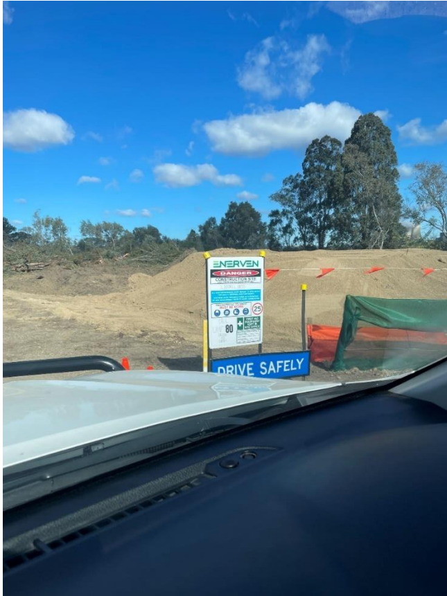
Plate 11 Signage situated at the entrance of Area 2, Stage 2 indicating speed limits
