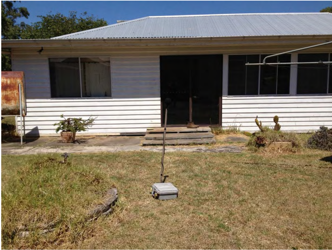
Figure 25 View to South at T25A
