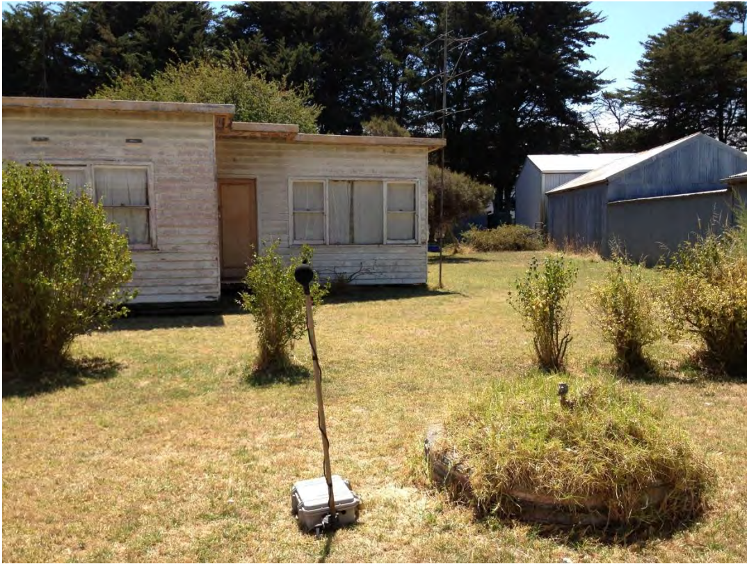
Figure 23 View to North at T25A
