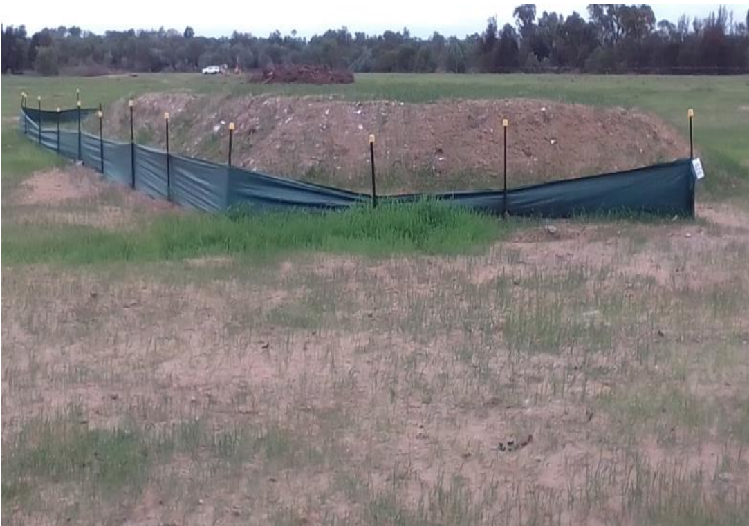
Plate 14 Stockpiles located within the Stage 2 site
