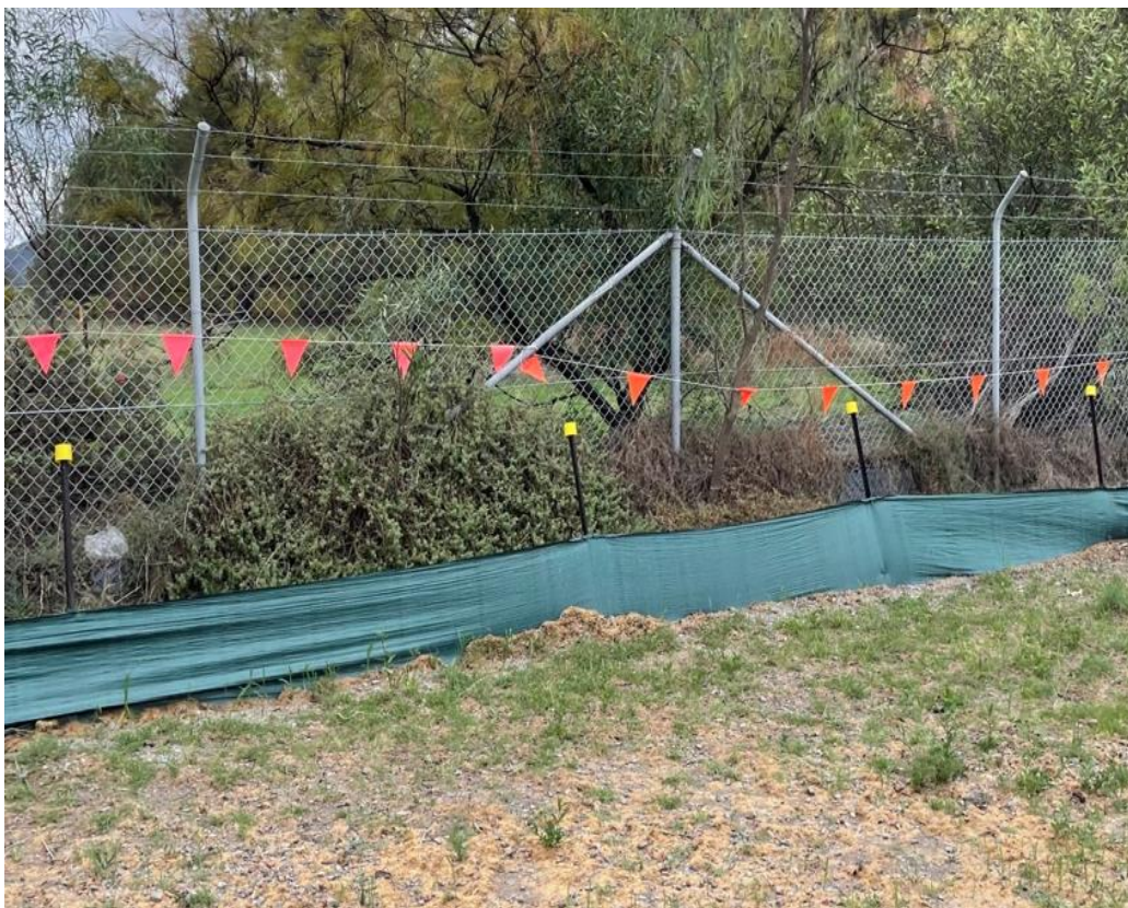
Plate 12 Sediment fencing and boundary flagging to delineate the Stage 2 site
