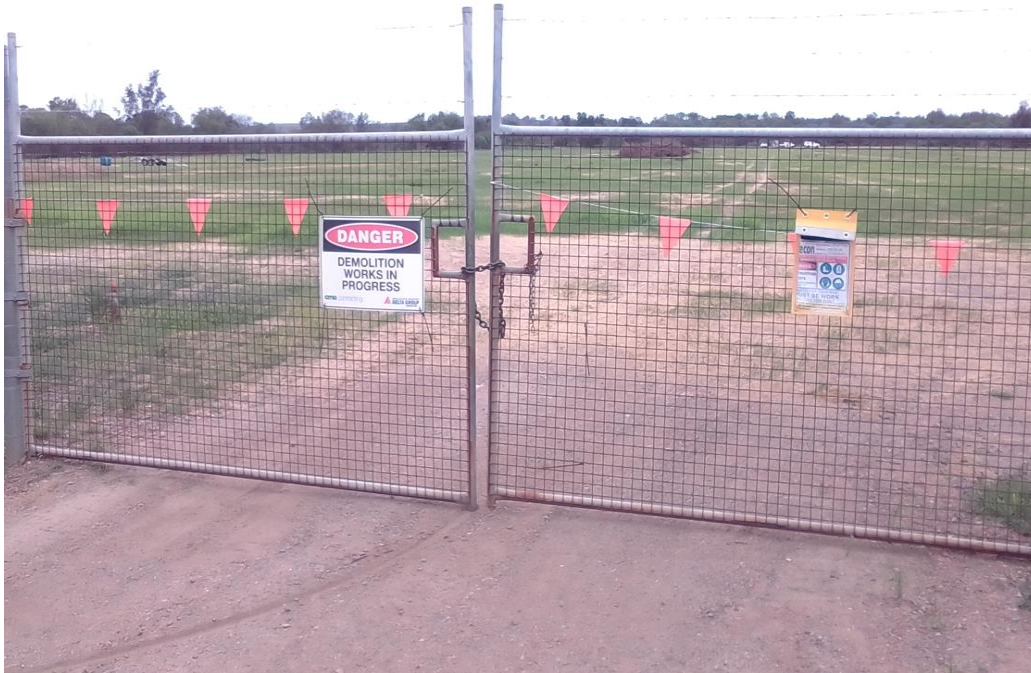
Plate 11 Locked gate and fencing surrounding the Stage 2 site
