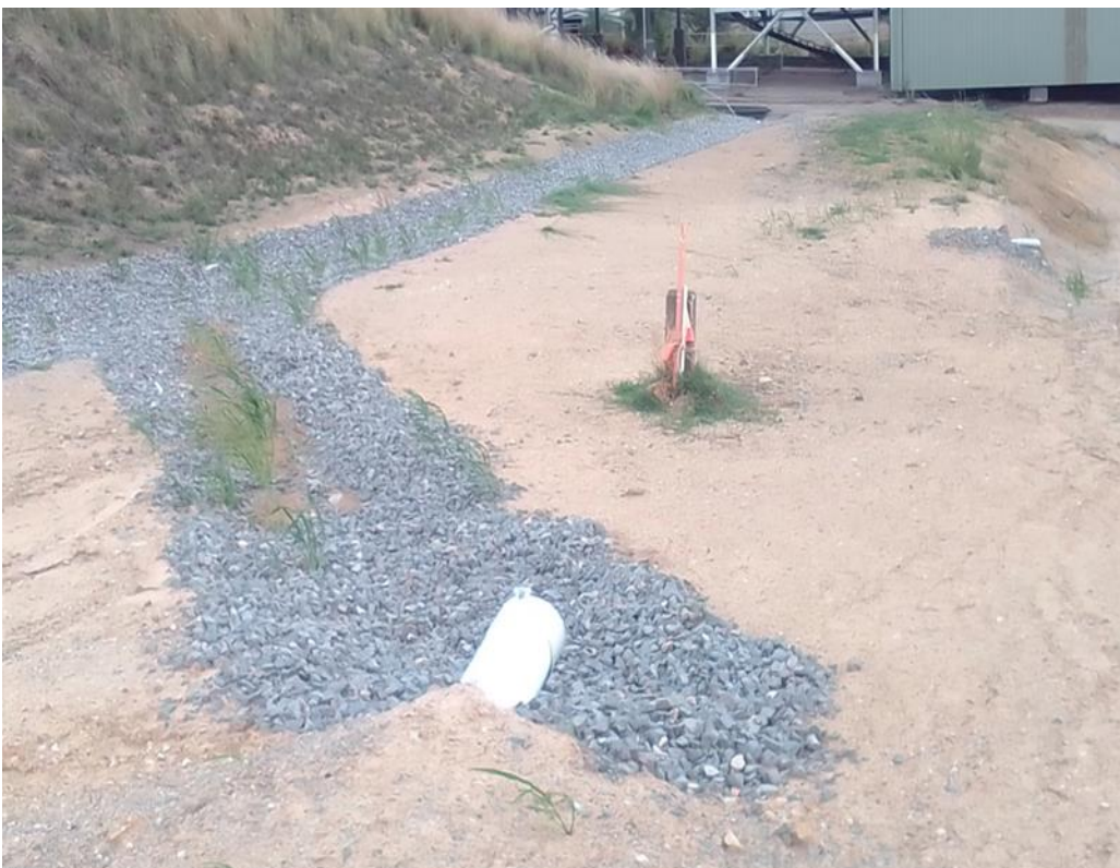
Plate 3 Erosion and sediment control measures available on the Stage 1 site
