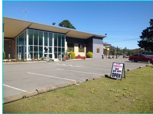
Tomago Bowling and Sporting Club 657 Tomago Rd, Tomago NSW 2322
