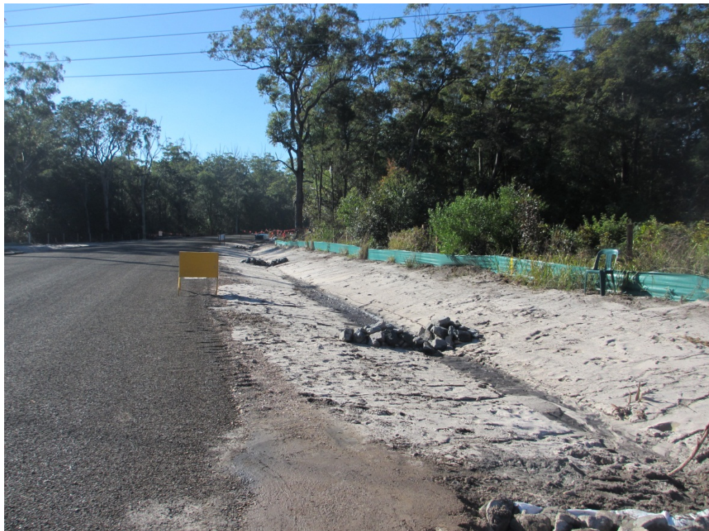
Figure 4.1 Silt fencing and rock checks installed along Main Access Road
