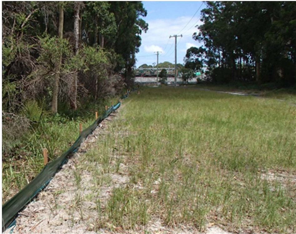
Photograph 4.1 Silt fencing installed along the Ausgrid easement
