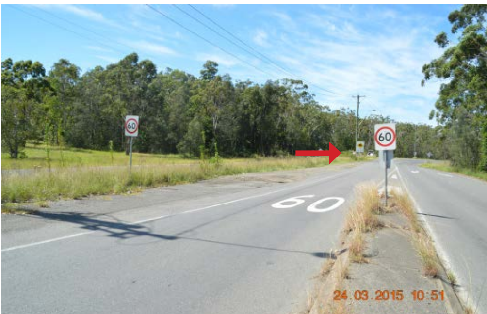
Speed signs on Old Punt Road near the intersection.
