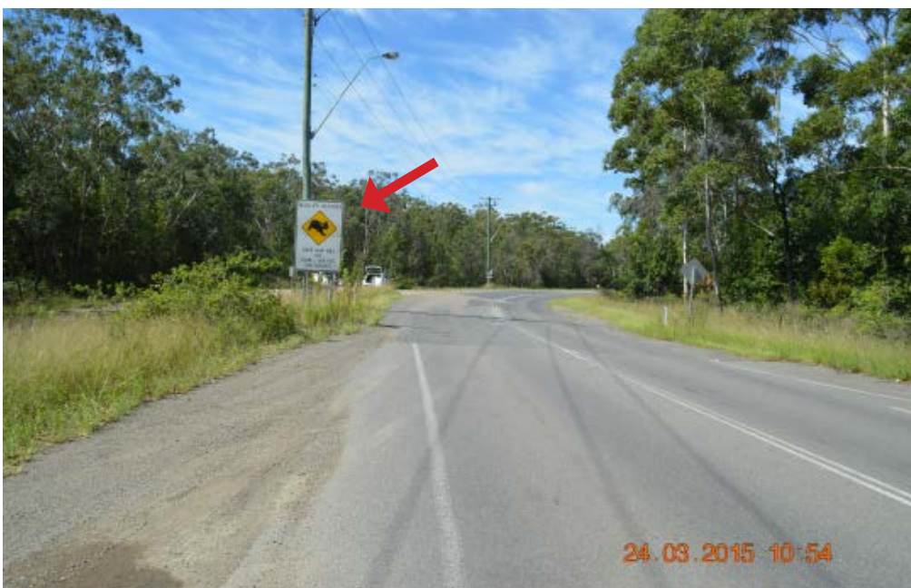
North side of Old Punt Road at 90 metres from the intersection with the Pacific Highway.
