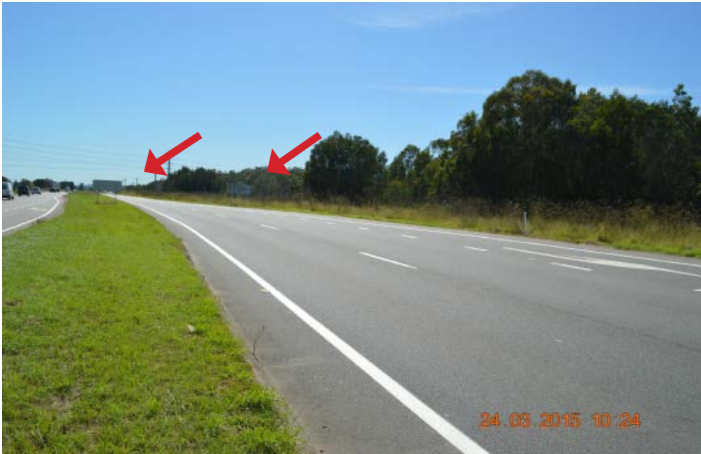
East side of Pacific Highway at 80 metres to the north of the intersection with Old Punt Road.
