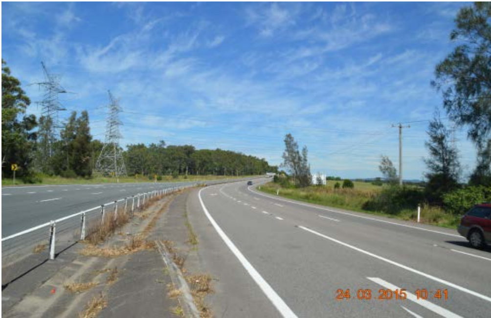
General view of the west side of the Pacific Highway at 140 metres to the south of the 'Slippery When Wet' street sign on the north side of the intersection with Old Punt Road.
