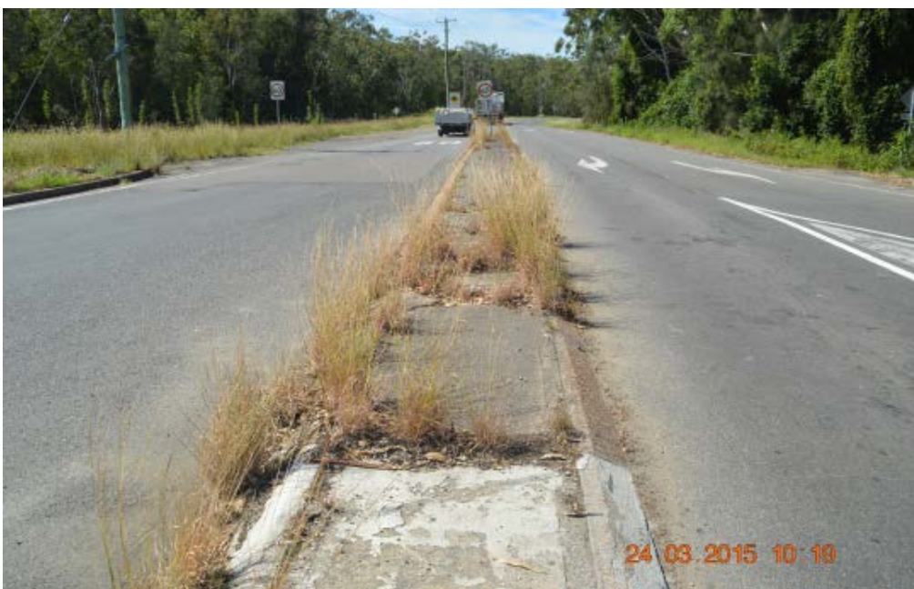
General view of Old Punt Road at the intersection with Pacific Highway.
