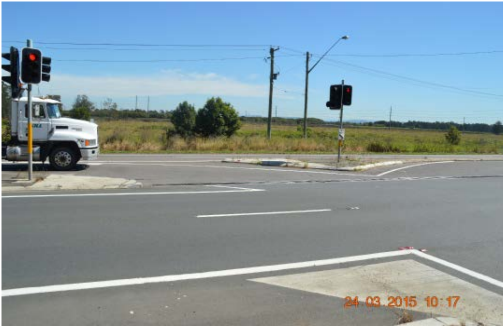
General view of Pacific Highway at the intersection with Old Punt Road.
