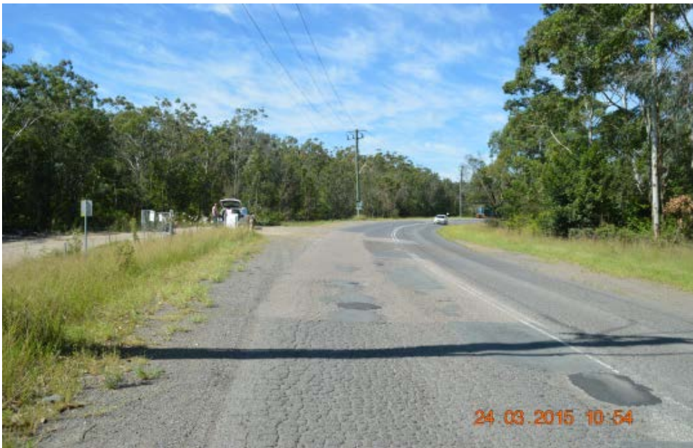
North side of Old Punt Road at 110 metres from the intersection with the Pacific Highway.
