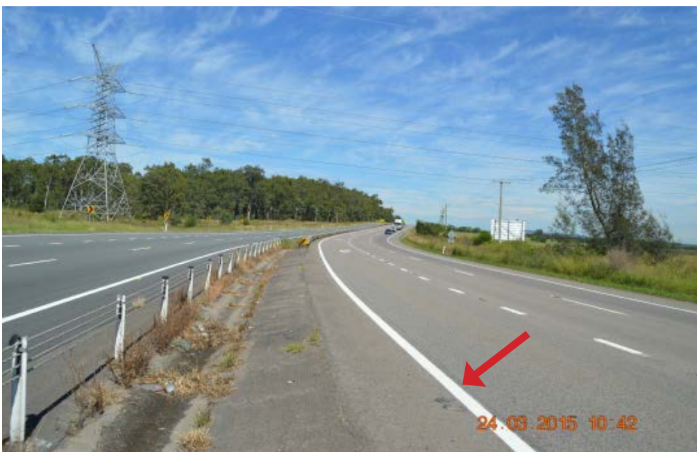
General view of the west side of the Pacific Highway at 190 metres to the south of the 'Slippery When Wet' street sign on the north side of the intersection with Old Punt Road.
