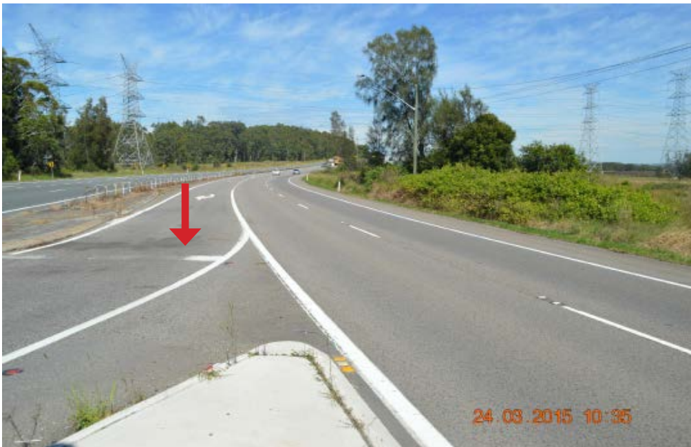
General view of the west side of the Pacific Highway at 110 metres to the south of the 'Slippery When Wet' street sign on the north side of the intersection with Old Punt Road.
