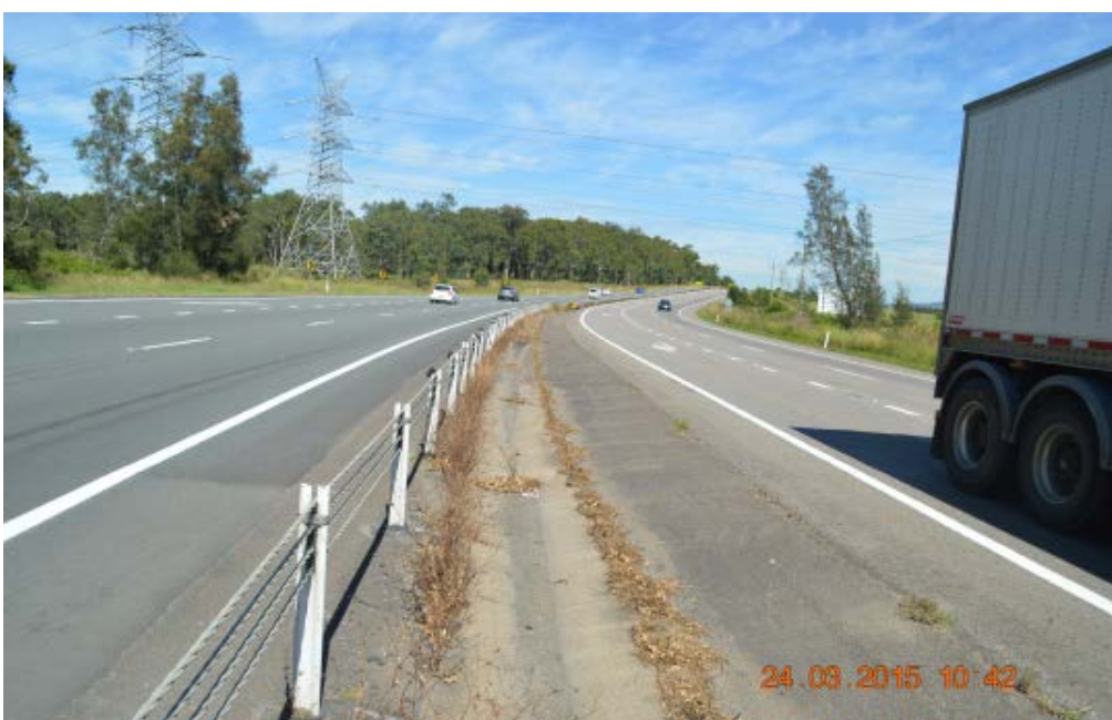
General view of the west side of the Pacific Highway at 160 metres to the south of the 'Slippery When Wet' street sign on the north side of the intersection with Old Punt Road.
