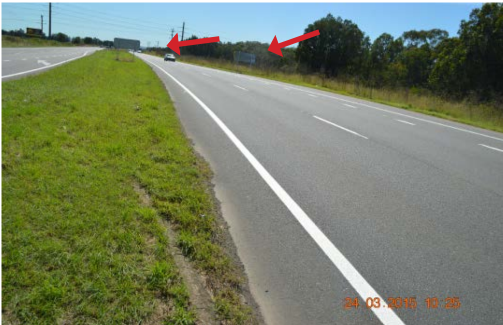
East side of Pacific Highway at 90 metres to the north of the intersection with Old Punt Road.
