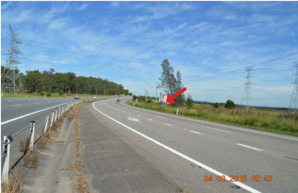
General view of the west side of the Pacific Highway at 170 metres to the south of the 'Slippery When Wet' street sign on the north side of the intersection with Old Punt Road.
