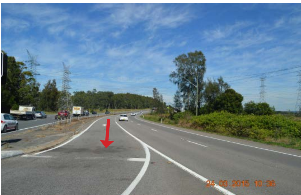
General view of the west side of the Pacific Highway at 110 metres to the south of the 'Slippery When Wet' street sign on the north side of the intersection with Old Punt Road.
