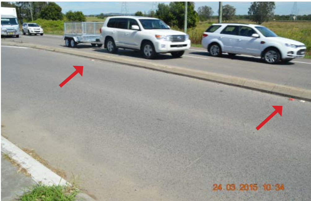
General view of the west side of the Pacific Highway at 80 metres to the south of the 'Slippery When Wet' street sign on the north side of the intersection with Old Punt Road.
