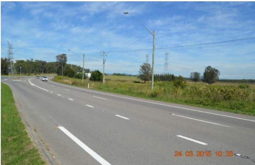
General view of the west side of the Pacific Highway at 40 metres to the south of the 'Slippery When Wet' street sign on the north side of the intersection with Old Punt Road.
