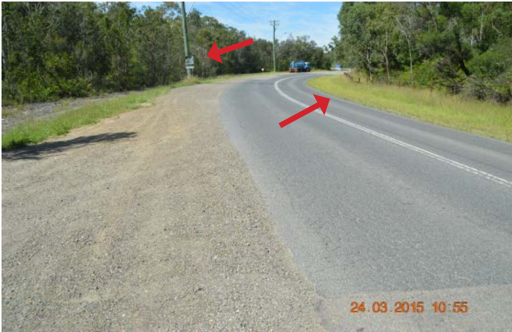
North side of Old Punt Road at 160 metres from the intersection with the Pacific Highway.
