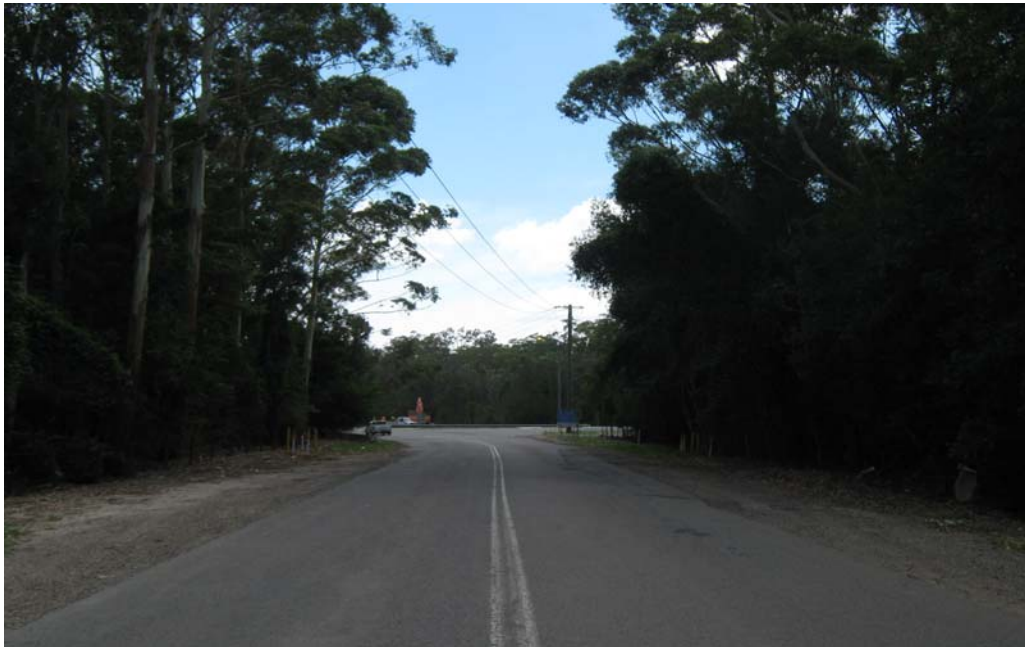
PHOTO P38 View north along Old Punt Road towards T Junction with Northern Access Road to Tomago Shelter.
