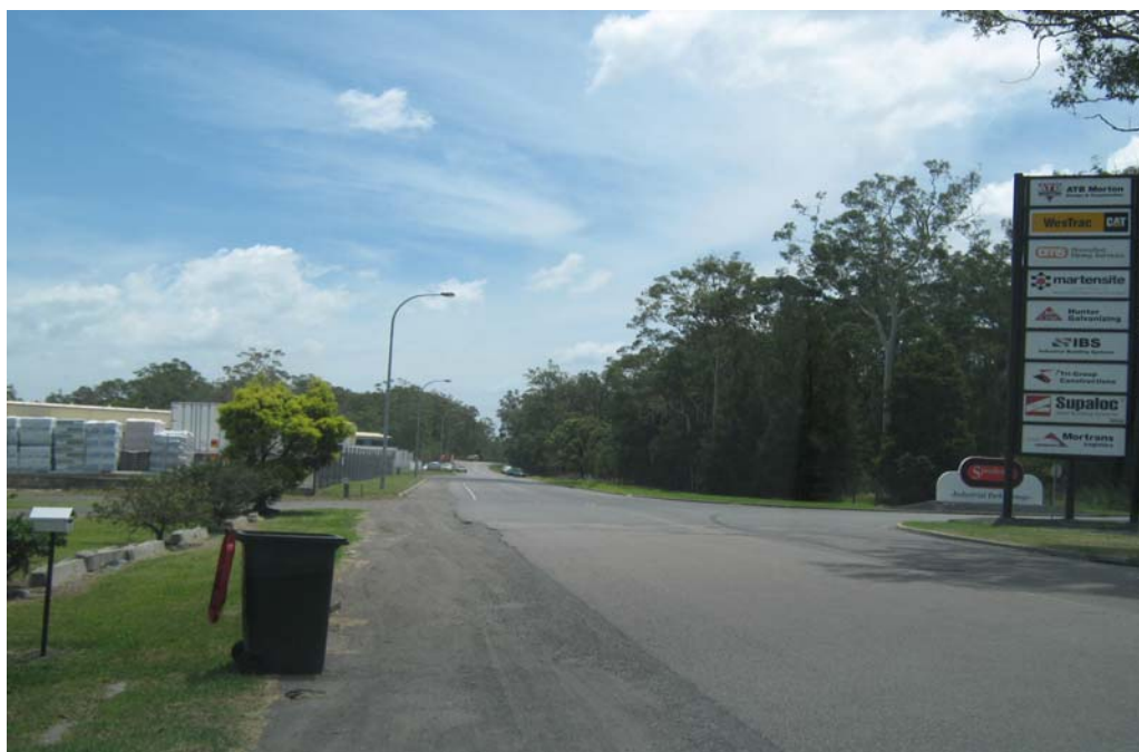
PHOTO P27 View North in Old Punt Road from point South of Industrial Estate Road.
