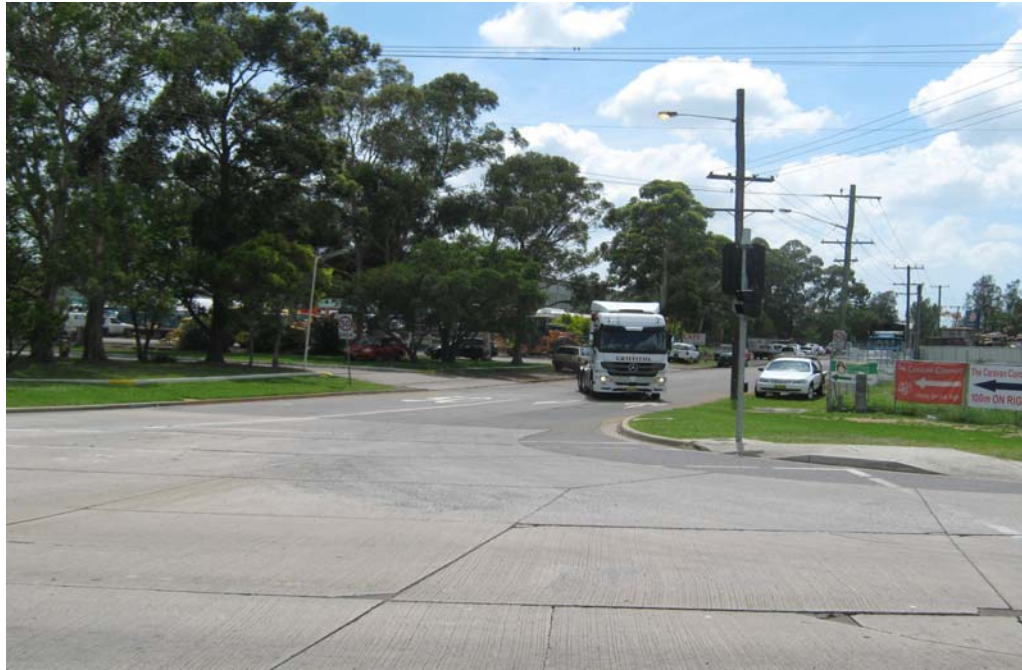
PHOTO P7 View of Old Maitland Road from Pacific Highway
