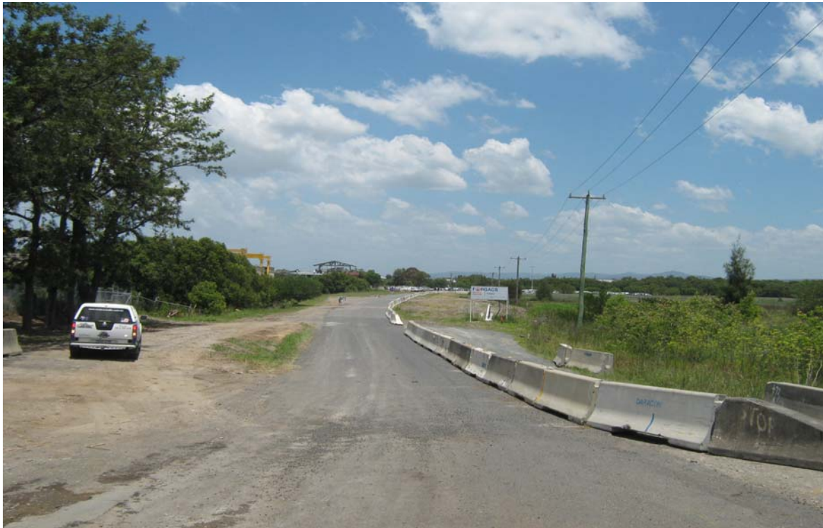
PHOTO P57 View South Along Old Punt Road Towards Hunter River from Laverick Avenue. Pipe Storage Area on Right of Concrete Barrier.
