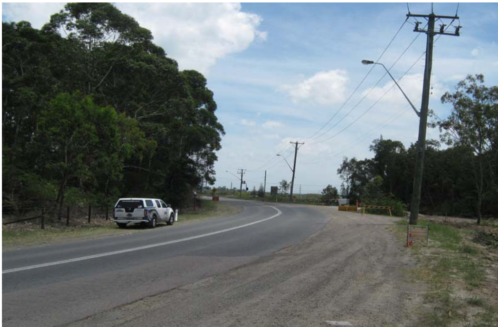
PHOTO P42 View west in Old Punt Road, NGSF Gravel access track (Junction) to Gas Storage Facility on right. Advance T Junction sign on left.
