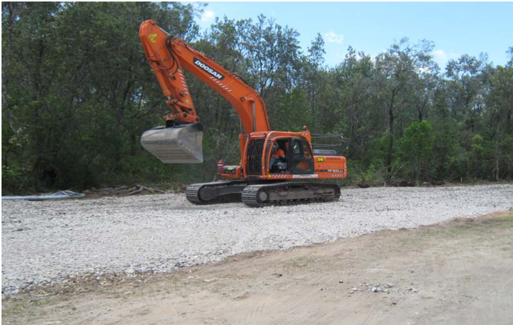
PHOTO P44 Stone Platform for Site 3 being prepared.
