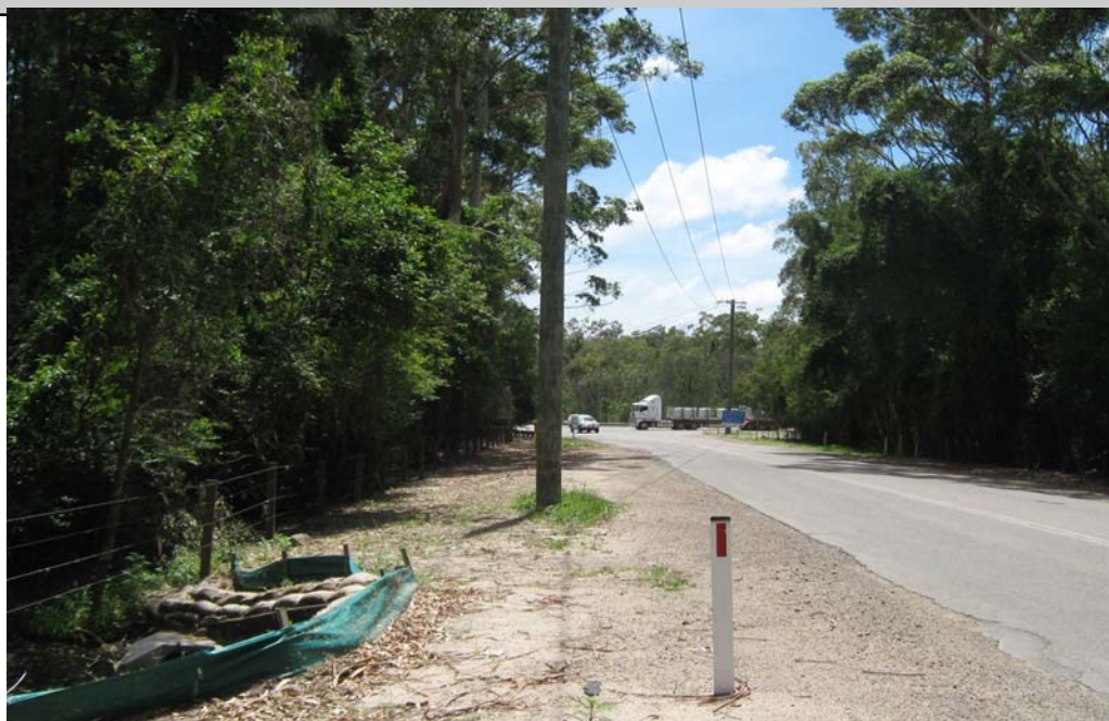
PHOTO P39 View north in Old Punt Road. Power Pole in Clear Zone.
