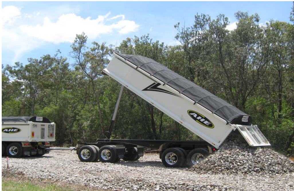
PHOTO P50 Truck/Trailer unloading stone ballast at Site 3.
