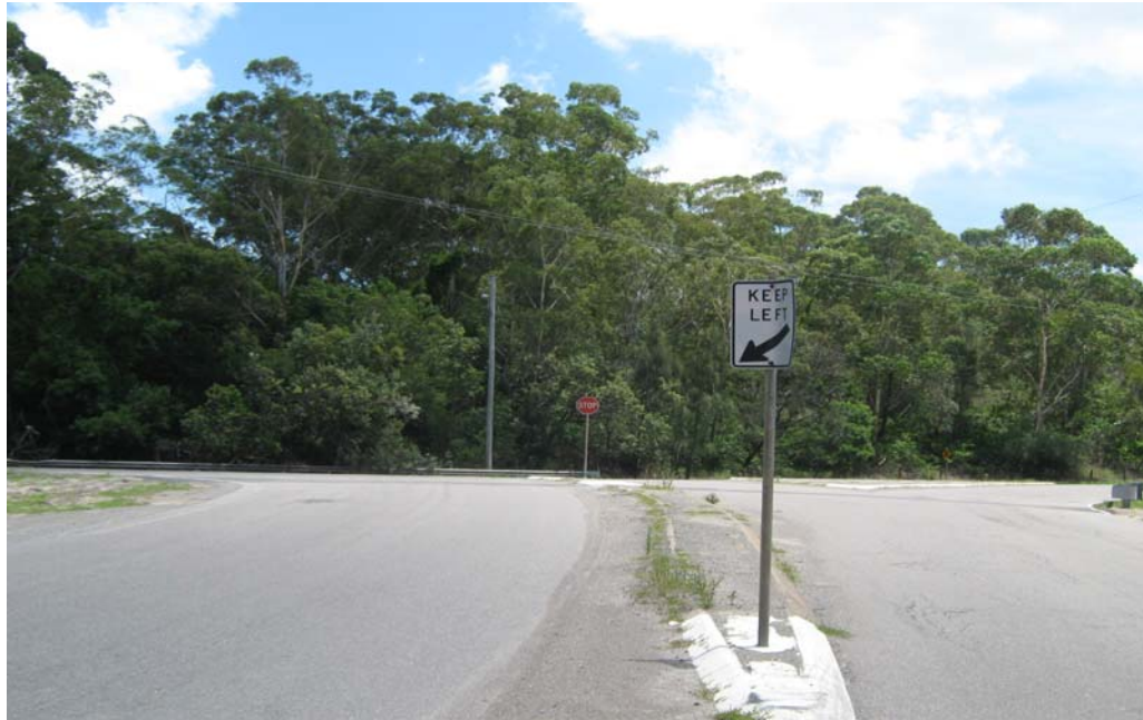
PHOTO P49 View west along Smelter access road towards channelised Junction with Old Punt Road.
