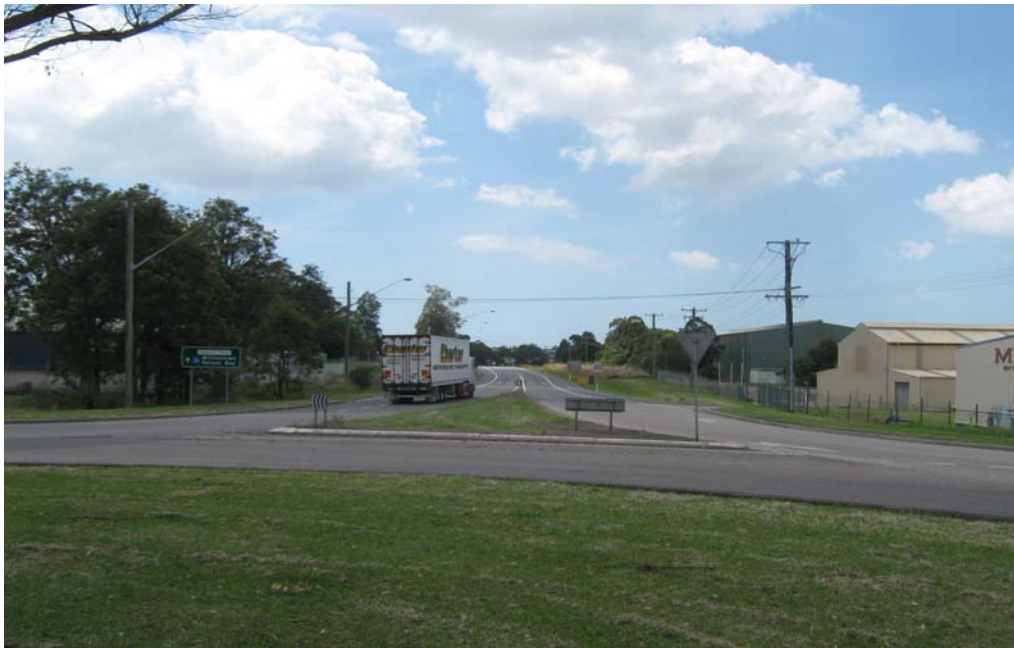
PHOTO P18 View of Southern leg of Roundabout at Tomago Road from Central Island.
