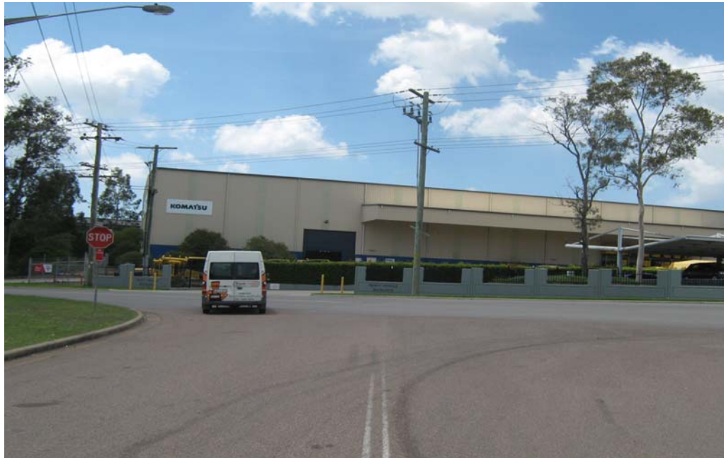
PHOTO P24 View East from Martin Drive to Old Punt Road
