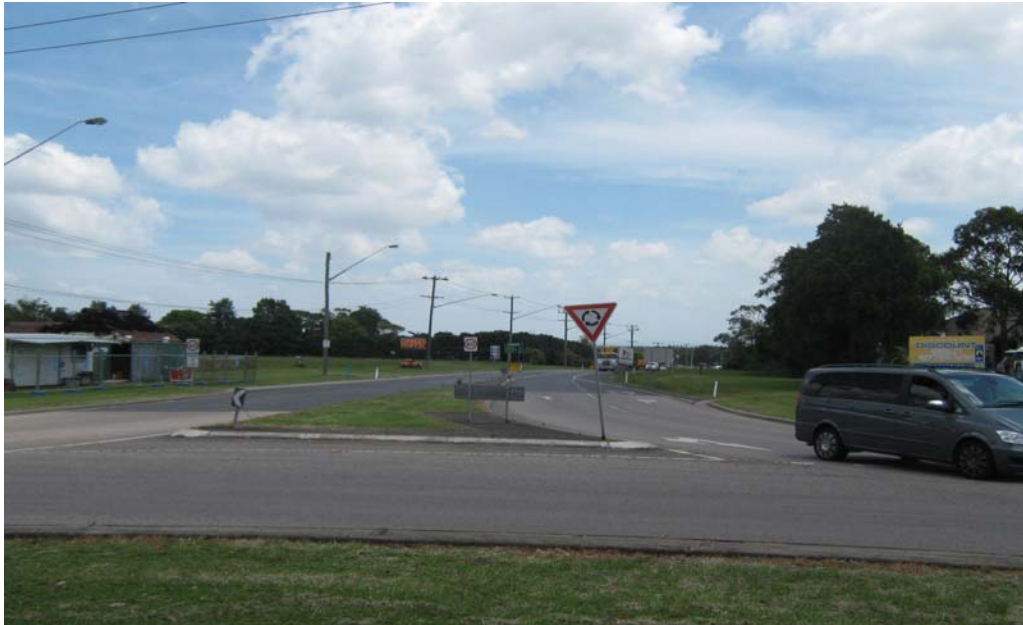
PHOTO P16 View of Southern leg of Roundabout at Tomago Road from Central Island.
