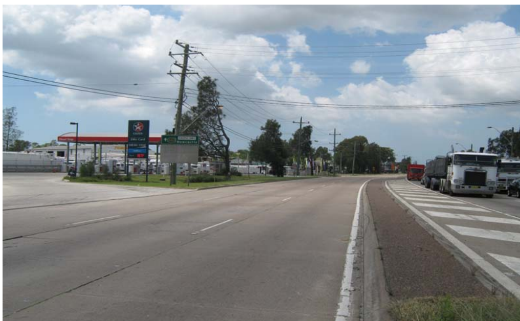
PHOTO P6 View East Along Pacific Highway at Old Maitland Road.
