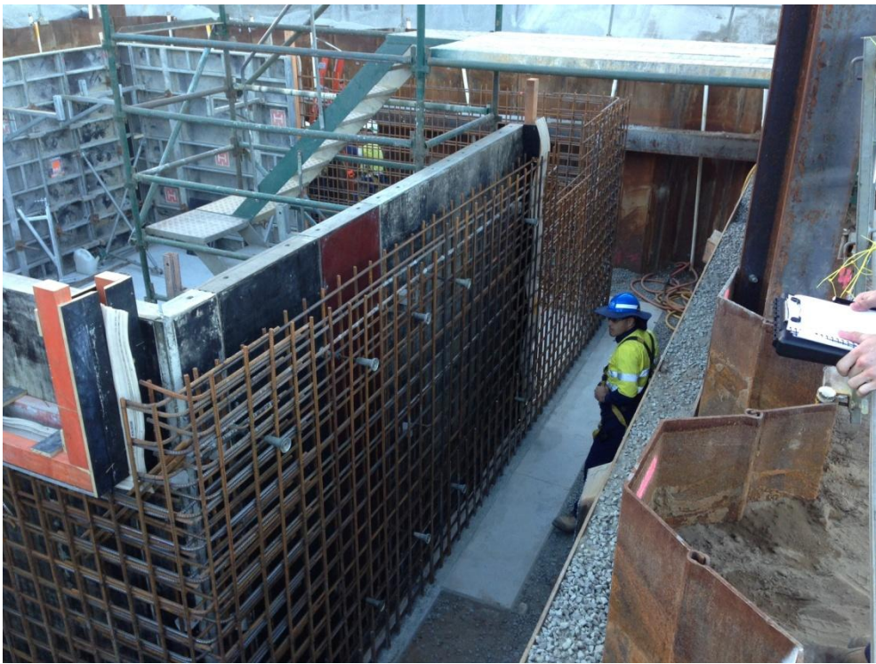
Photo showing installation of reinforcement.
