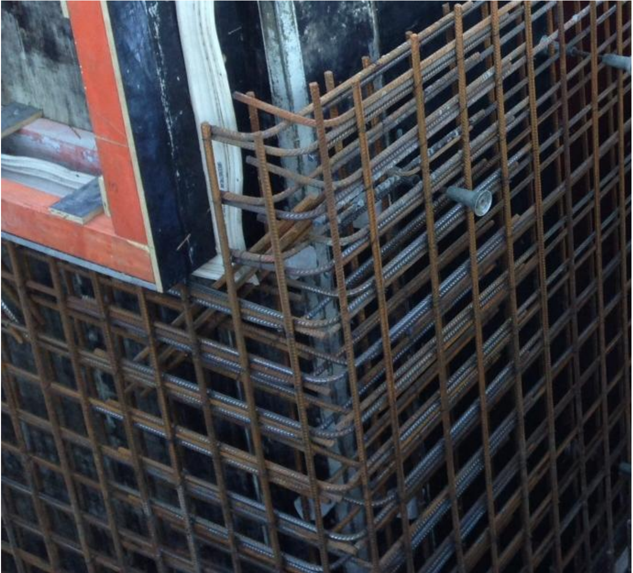
Corner reinforcement
