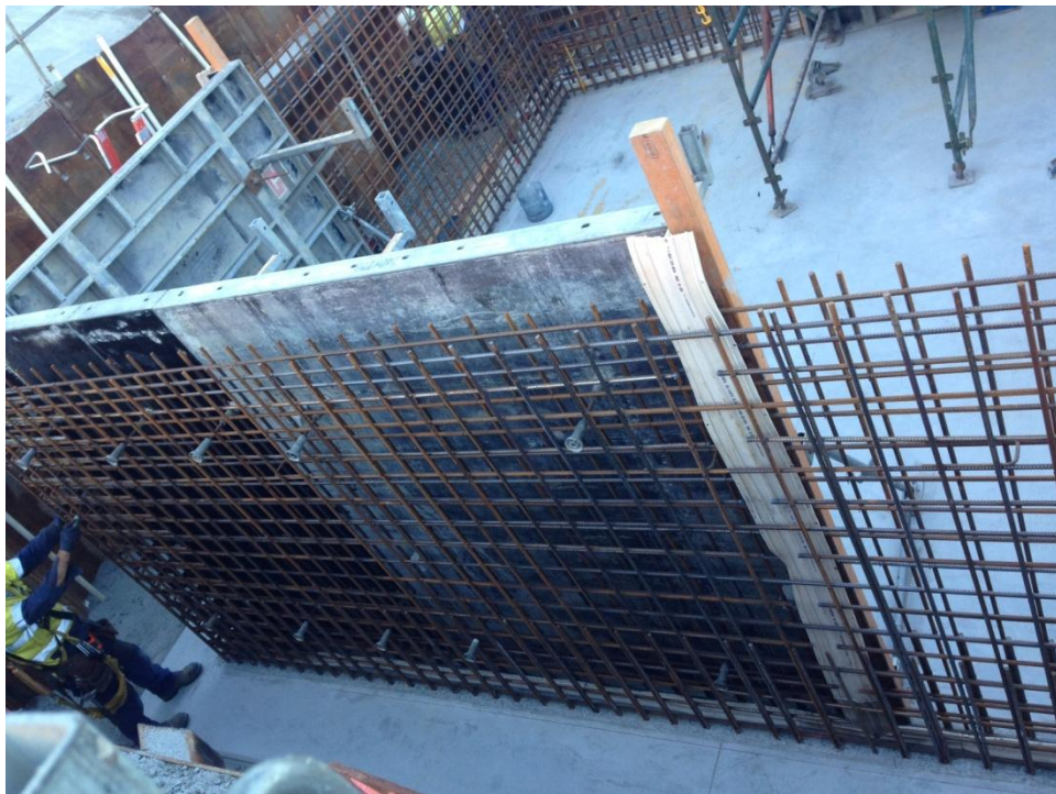
Waterstop located in side wall
