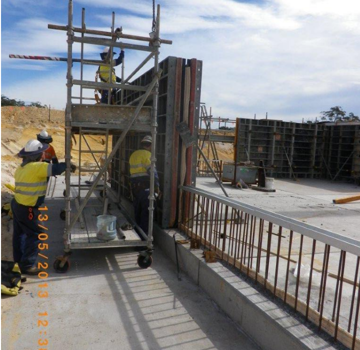
Note clean and tidy work area
