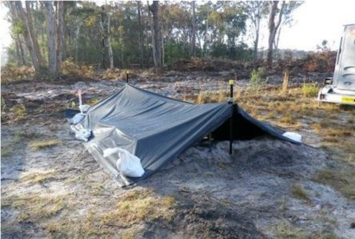
Generators bundled and sheltered from Rainfall and upslope runoff
