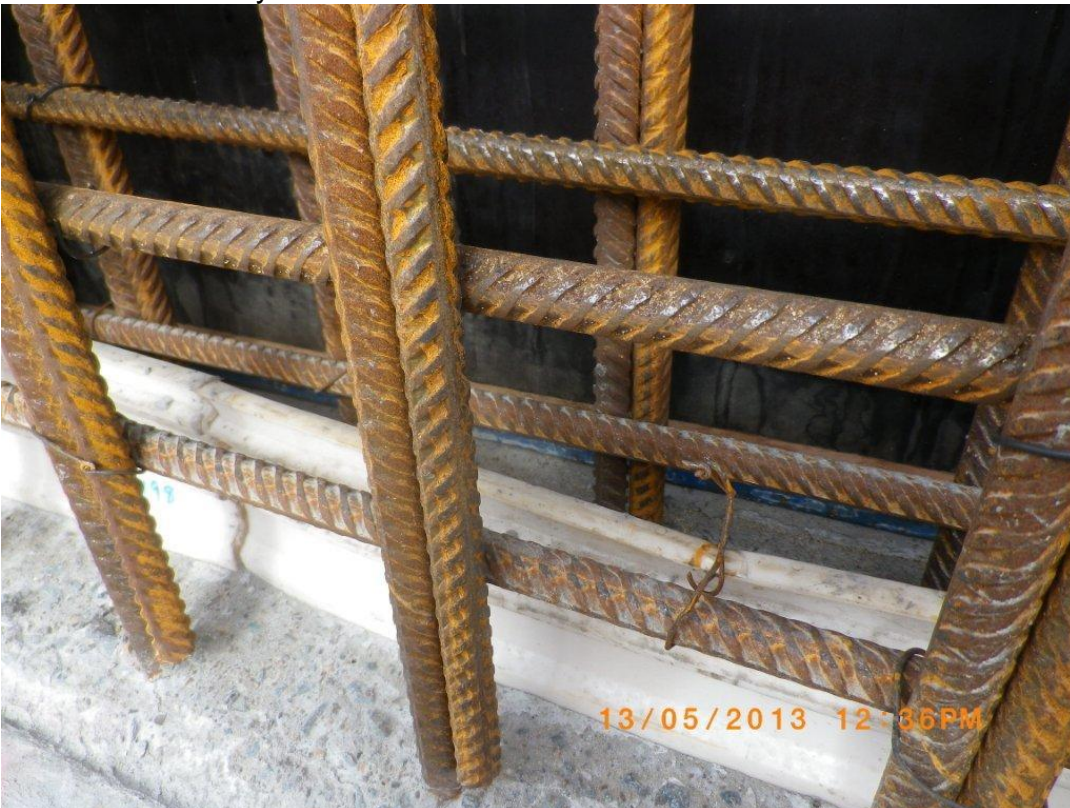
Water stop and adequate splicing of reinforcement
