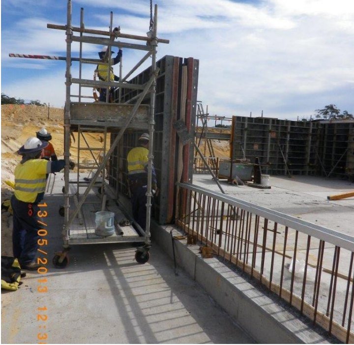
Note clean and tidy work area
