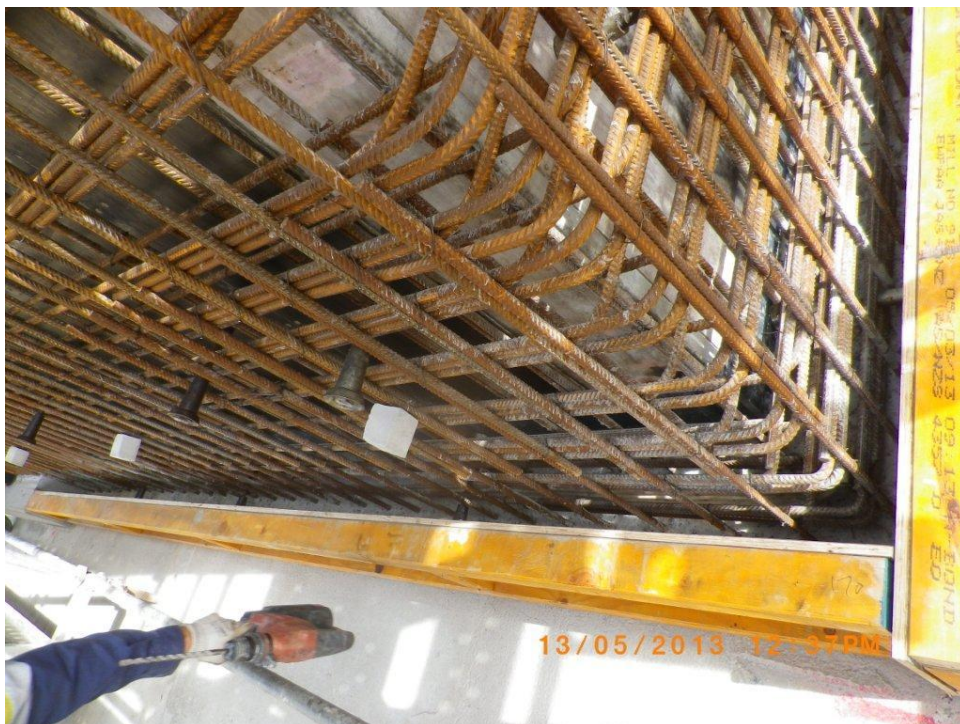
Correct detailing of reinforcement at corners
