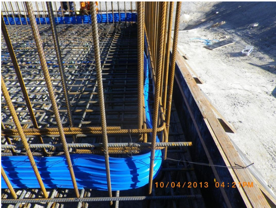
Waterstop in Wall – Note significant blinding layer in background and generally clean work area.
