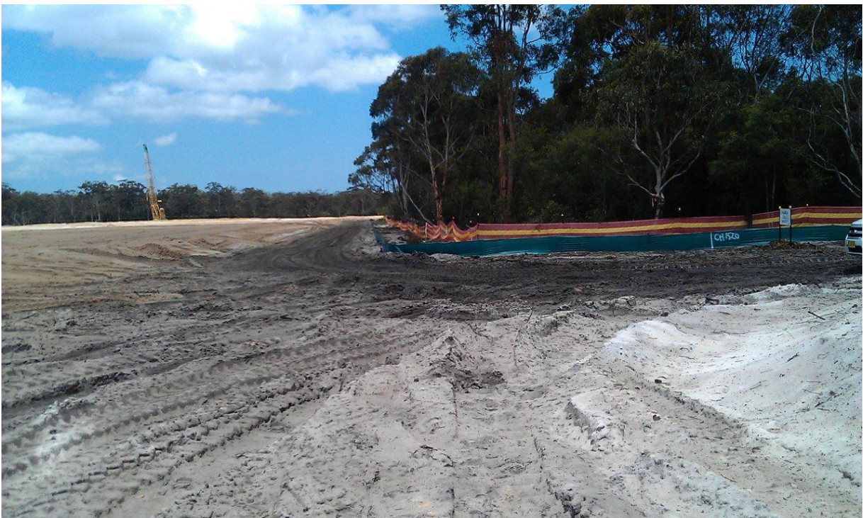
Sediment fence and barrier fencing
