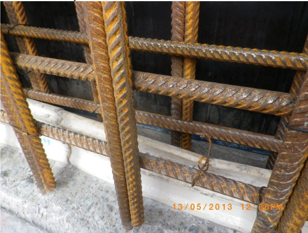
Water stop and adequate splicing of reinforcement
