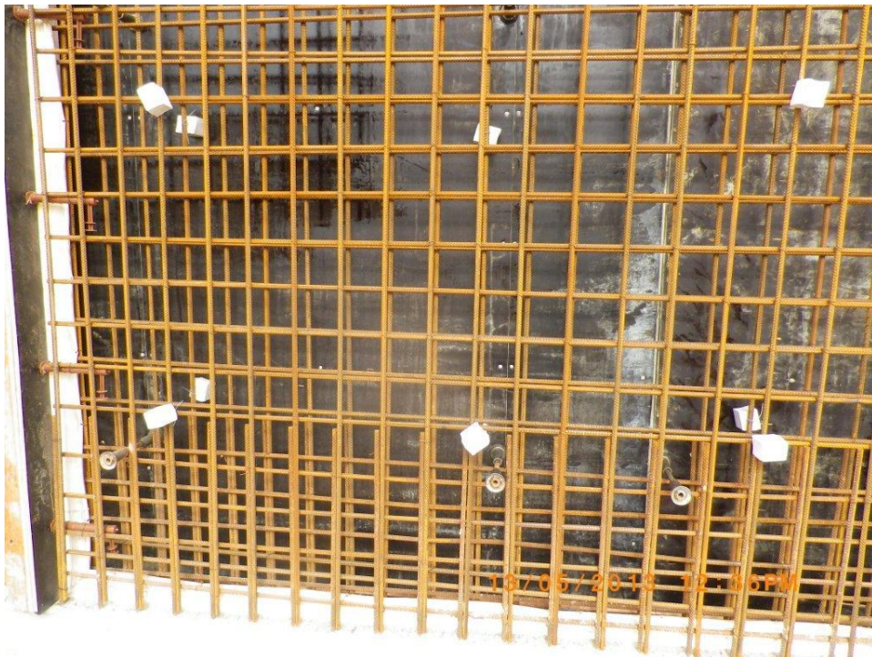
Waterstop at base and side of wall.
