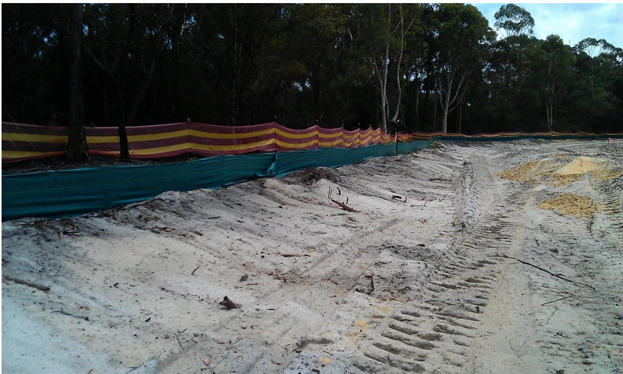
Sediment fence to perimeter of Site
