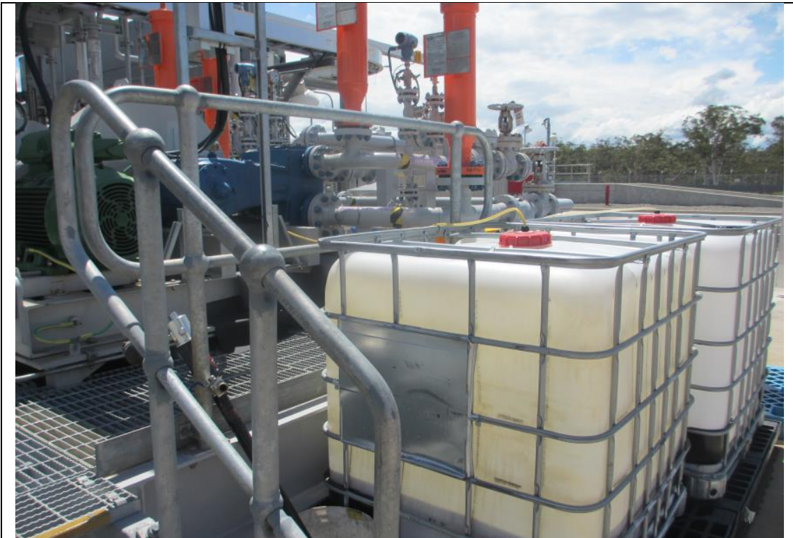
Photograph: 8 Amine leak from pump contained within IBCs which are stored on bund trays to contain any drips.
