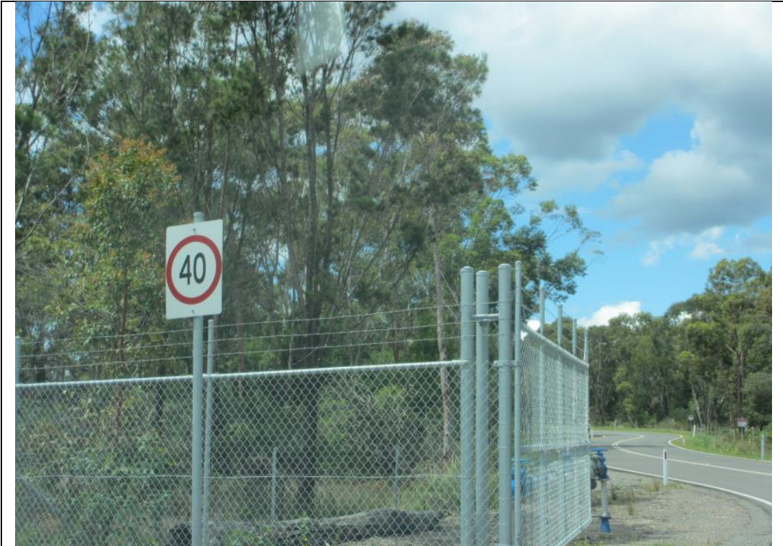
Photograph: 1 | Speed limit sign prior to bends in Main Access Road
