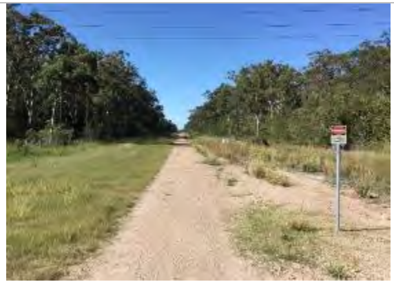
View of the road towards the east in SU6
