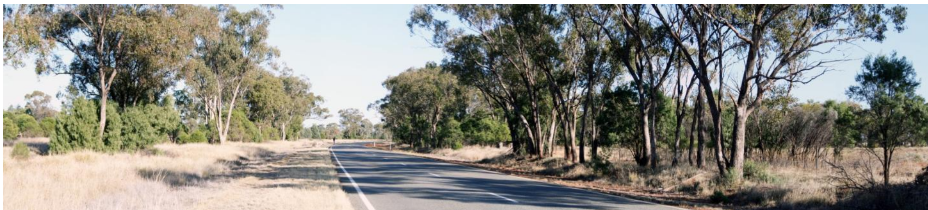
Existing conditions (above)
