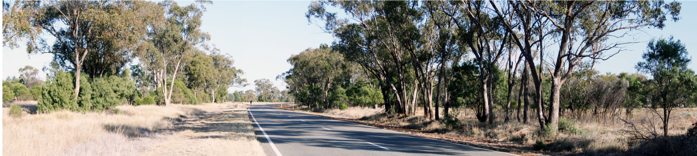
Existing conditions (above)
