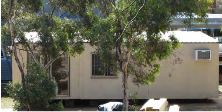
Figure 3.4 Typical prefabricated steel site office
