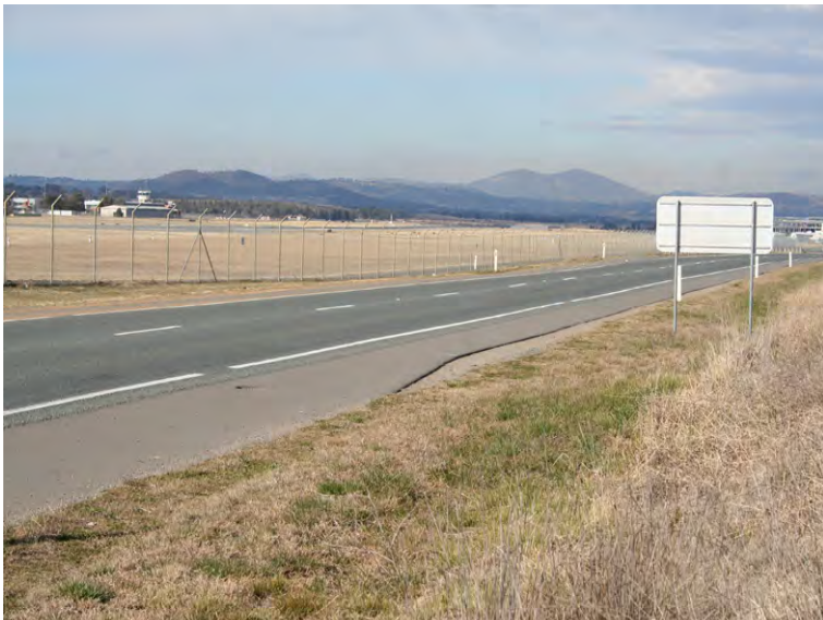
Figure 3.5 Example of site fence (top of posts may be straight instead of angled)
