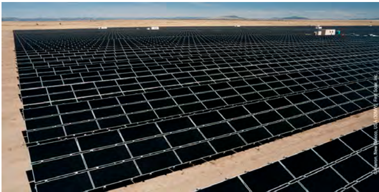
Figure 3.1 Typical solar arrays (image courtesy First Solar)
