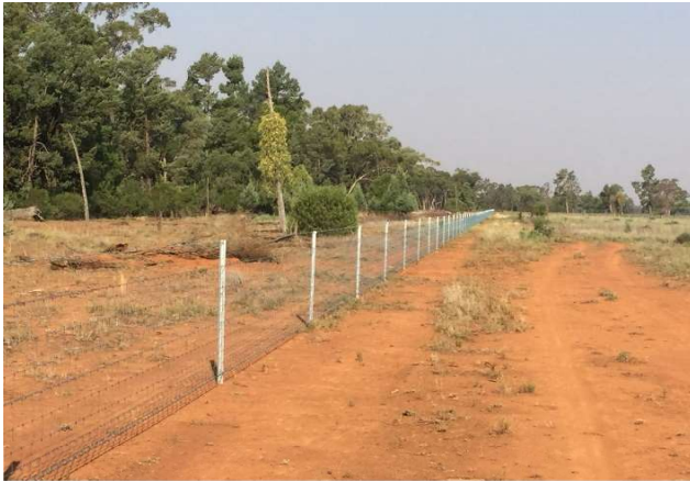
Plate 15 Ring-lock fencing with a top strand of barbed-wire along the southern boundary of the offset site. This style of fencing surrounds the entire perimeter of the offset site.
