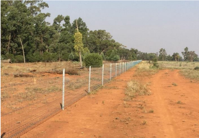
Photo 13 Ring-lock fencing along the southern boundary of the offset site. This style of fencing surrounds the entire perimeter of the offset site
