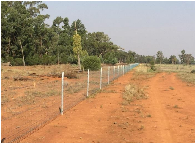
Plate 13 Ring-lock fencing along the southern boundary of the offset site. This style of fencing surrounds the entire perimeter of the offset site.
