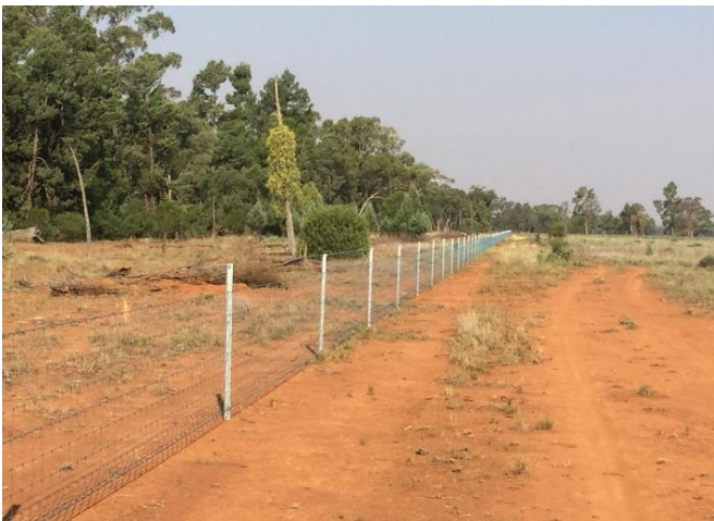
Plate 13. Ring-lock fencing along the southern boundary of the offset site. This style of fencing surrounds the entire perimeter of the offset site.
