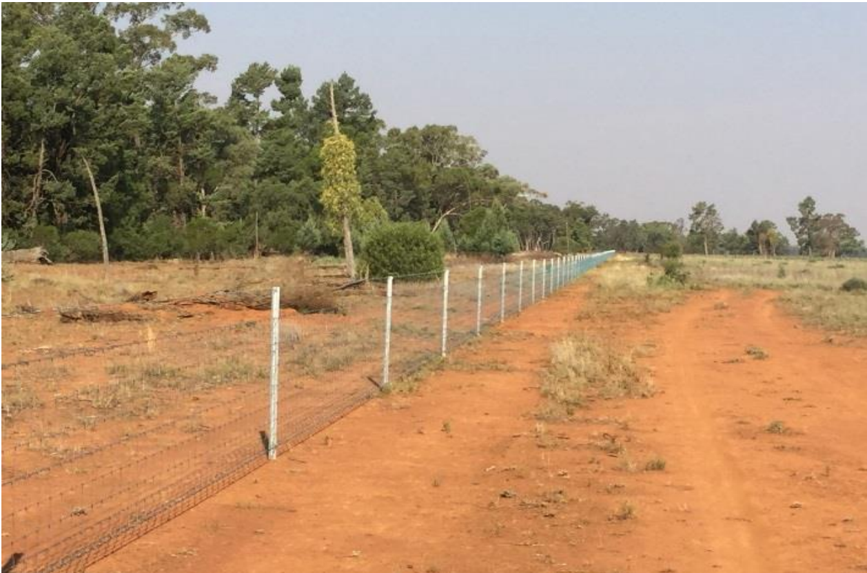
Plate 13. Ring-lock fencing along the southern boundary of the offset site. This style of fencing surrounds the entire perimeter of the offset site.
