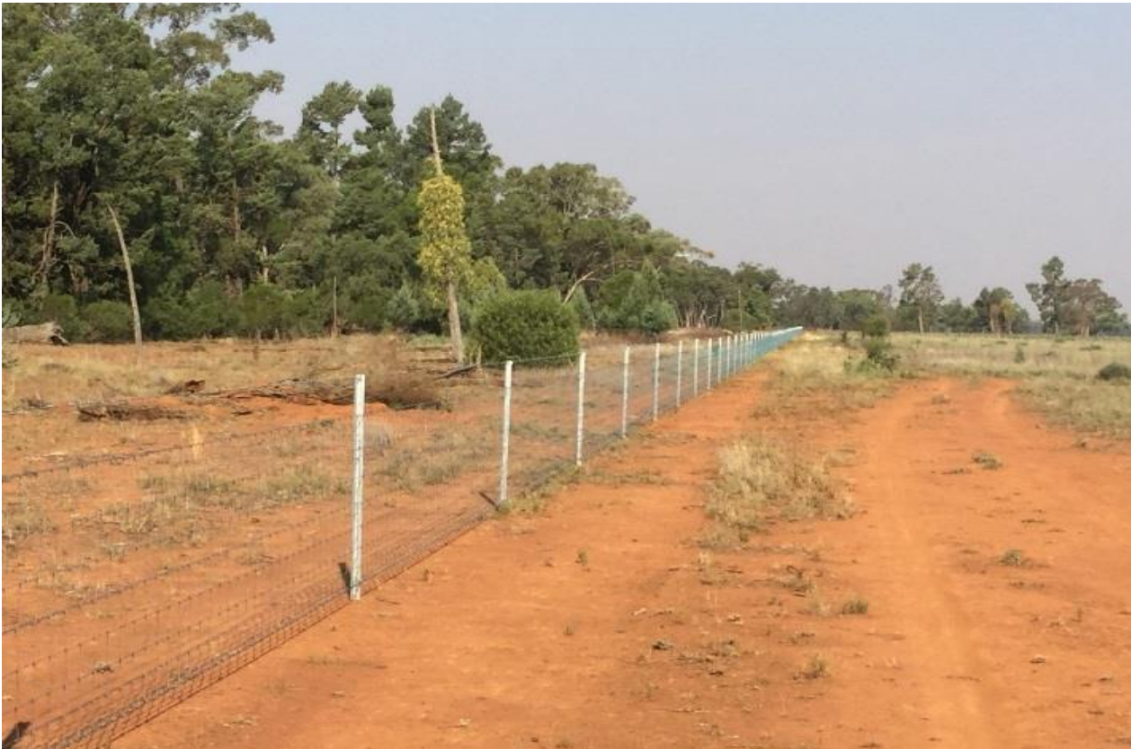
Plate 14. Ring-lock fencing along the southern boundary of the offset site. This style of fencing surrounds the entire perimeter of the offset site
