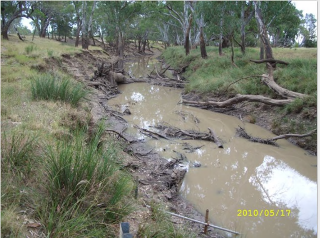
Stream gauging station 417205A – Moonie River at Flinton (Source: Qld Govt – Water Monitoring Information Portal).
