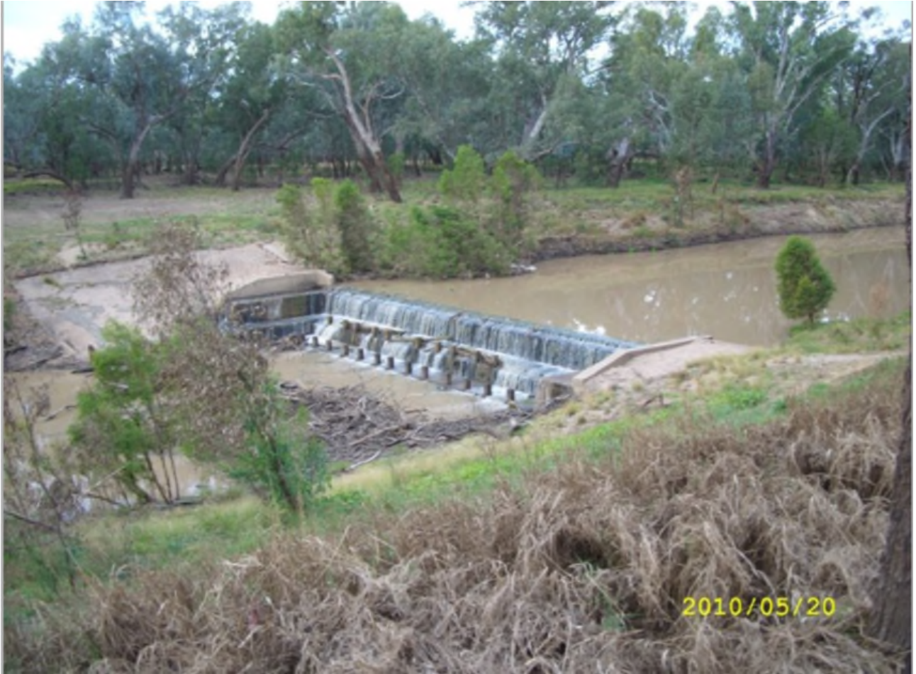
Stream gauging station 422220A - Balonne River at Surat (Source: Qld Govt - Water Monitoring Information Portal).
